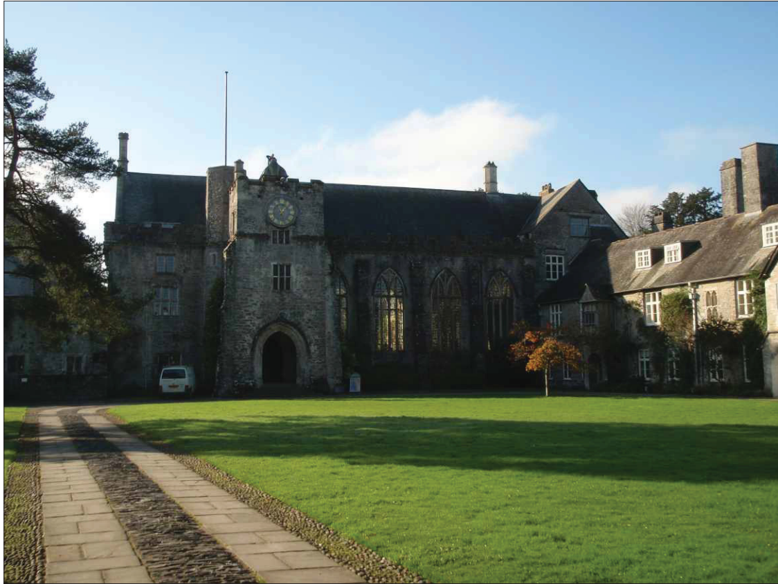
Plate 3: Dartington Hall (site B5), view to southwest
