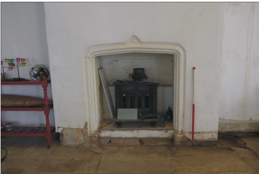
Plate 4: Fireplace, looking northwest (1m scale)
