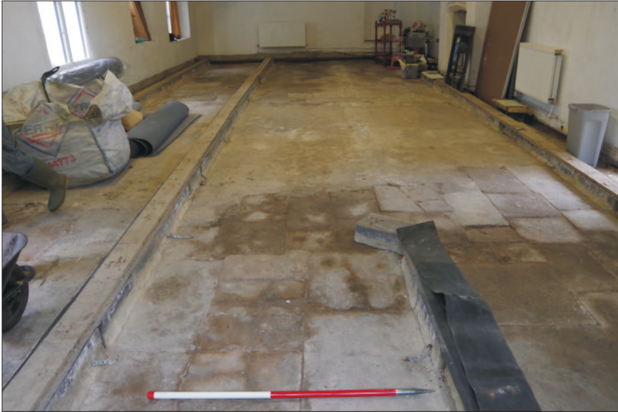
Plate 1: Floor prior to modern blockwork being removed, looking southwest (1m scale)
