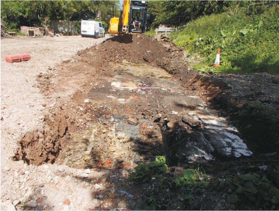
Plate 3: Trench 1, looking northeast (1m scale)
