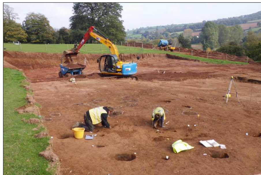
Plate 4: Structure 1, work in progress, looking ENE
