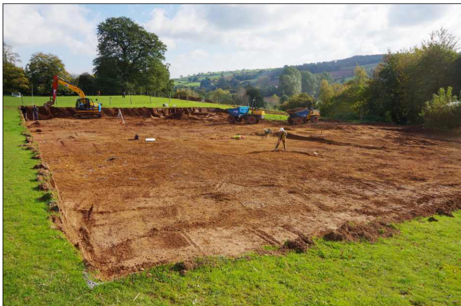
Plate 1: View of site, work in progress, looking southeast
