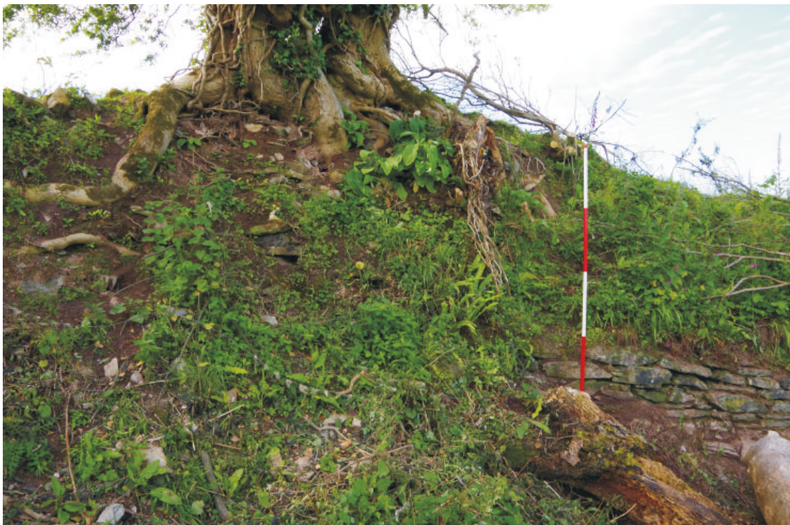
Plate 8: Zone 2, eastern corner of northwest wall, showing erosion cone, viewed from the north. 2m scale
