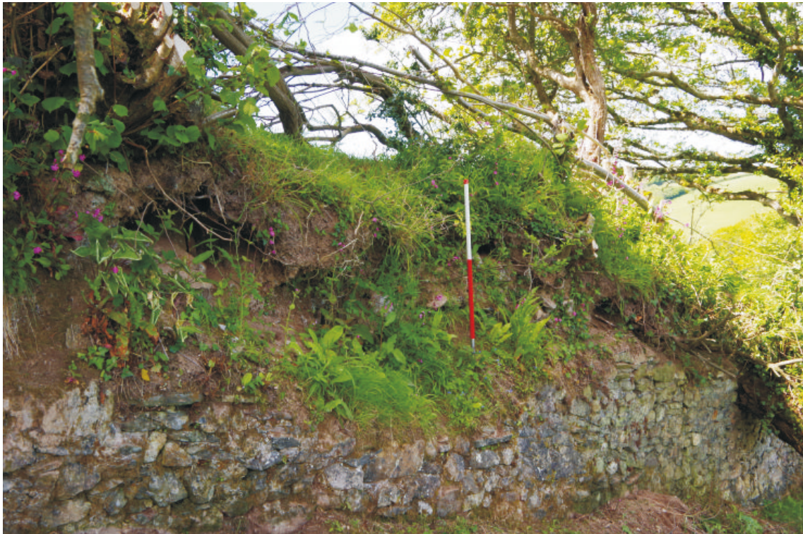
Plate 9: Zone 2, northwest wall, wild animal burrowing, viewed from the northeast. 1m scale
