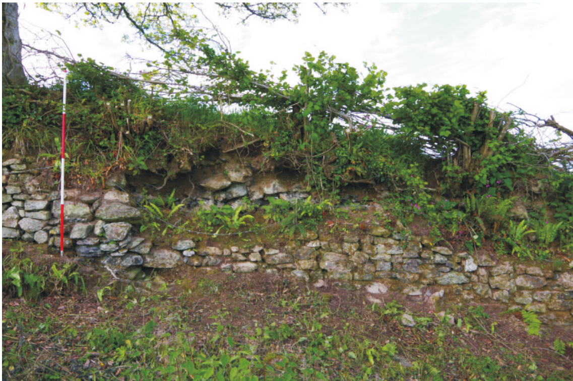
Plate 7: Zone 2, northwest wall, showing exposed core, viewed from the northwest. 2m scale
