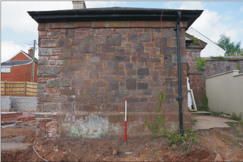
Plate 4: East elevation of the lodge, looking from the east (1m scale)
