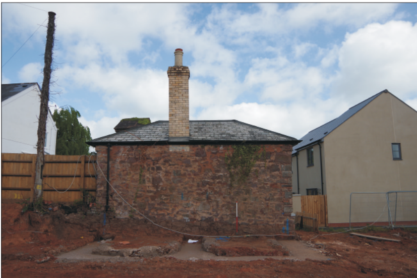
Plate 3: South elevation of the lodge, looking from the south (1m scale)
