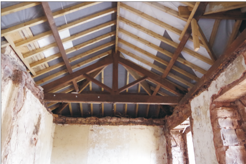
Plate 10: Roof truss in the lodge, looking from the east
