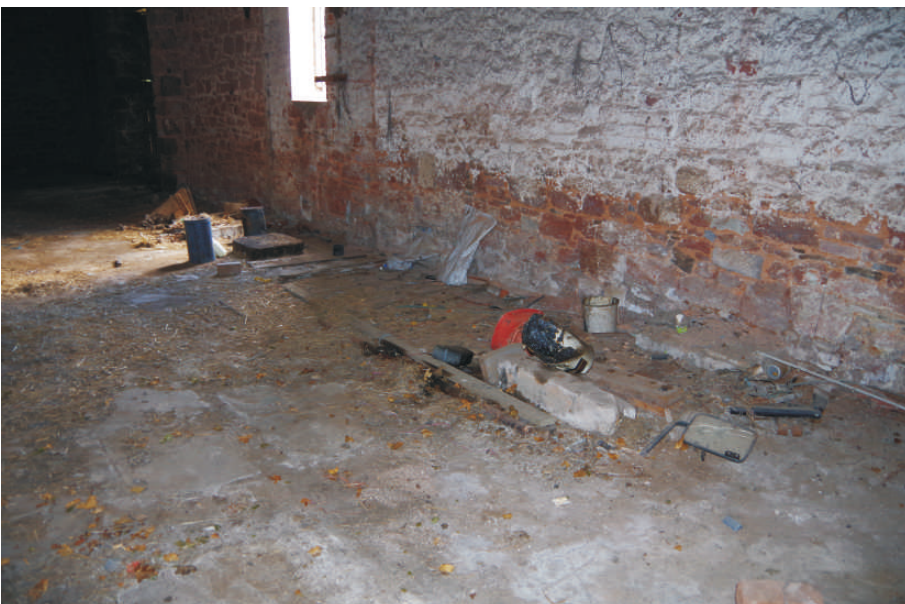
Plate 26: Concrete bases for machines in the northern end of the old barn, looking southwest
