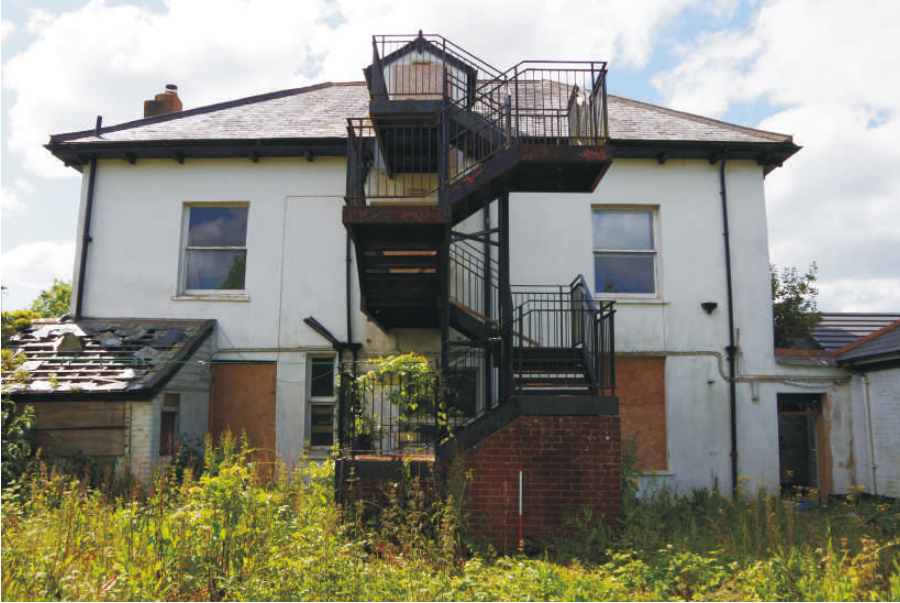
Plate 4: The north elevation of the house, looking south (1m scale)
