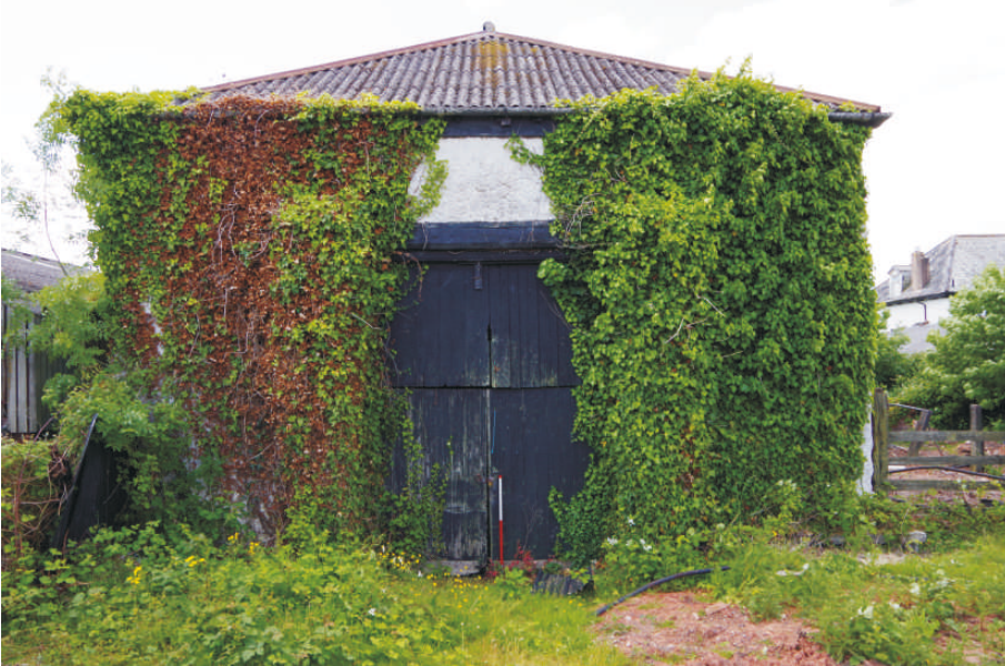
Plate 19: The north elevation of the old barn, looking south (1m scale)
