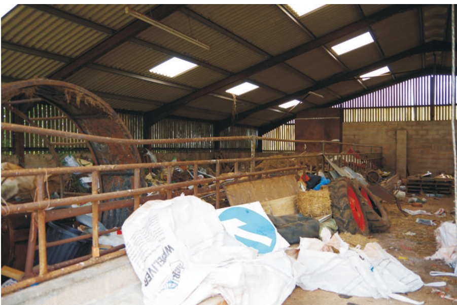
Plate 29: The new barn, looking south east
