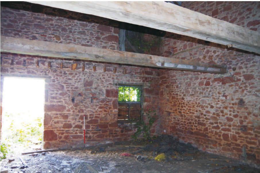
Plate 25: The southern end of the old barn, looking southeast (1m scale)
