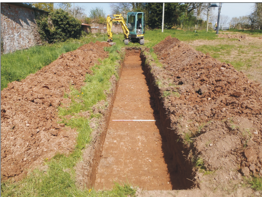
Plate 3: Trench 2, looking north (scale 1m)
