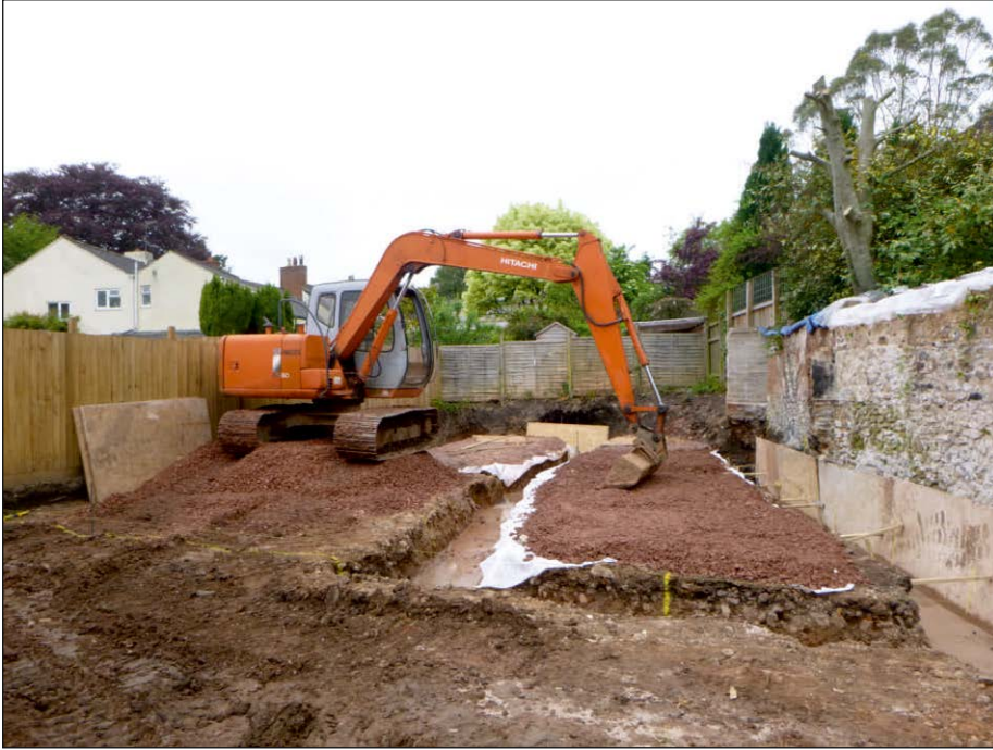
Plate 1: General working view of site, looking north
