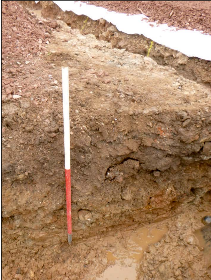
Plate 2: Representative view of footings trench. Looking north (scale 1m)
