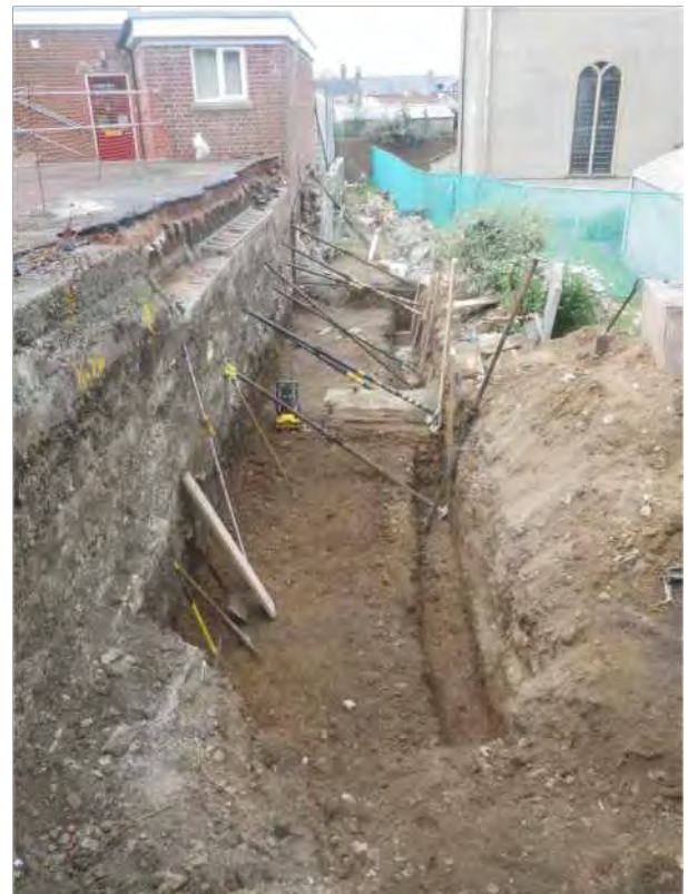
Plate 6: View of excavated trench, looking south
