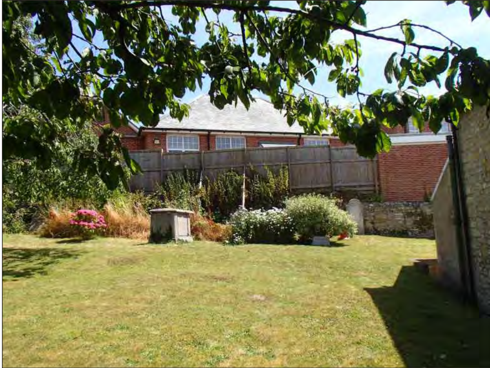
Plate 1: General view of graveyard and wall collapse, looking east
