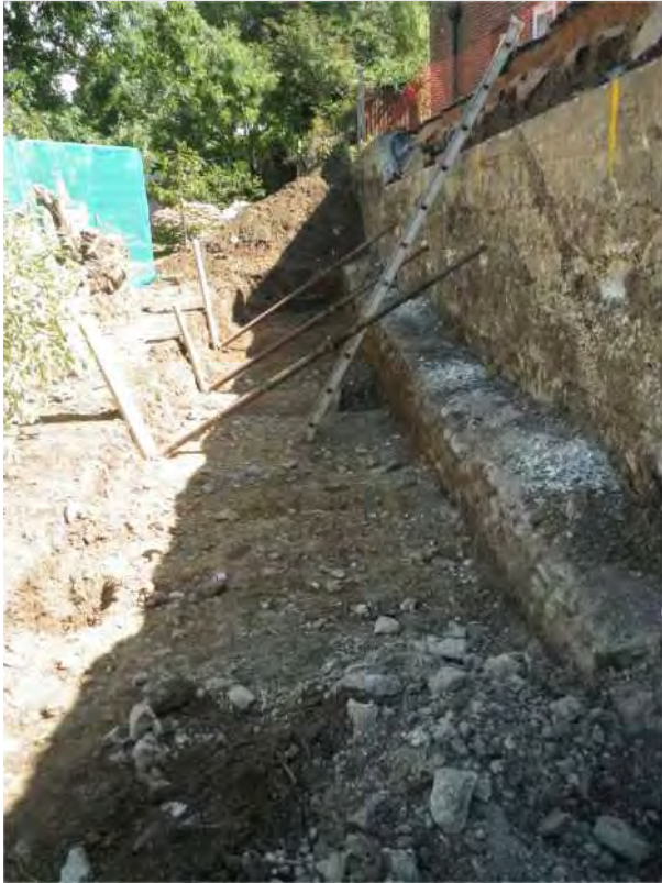
Plate 3: View of remaining boundary wall prior to removal, looking north
