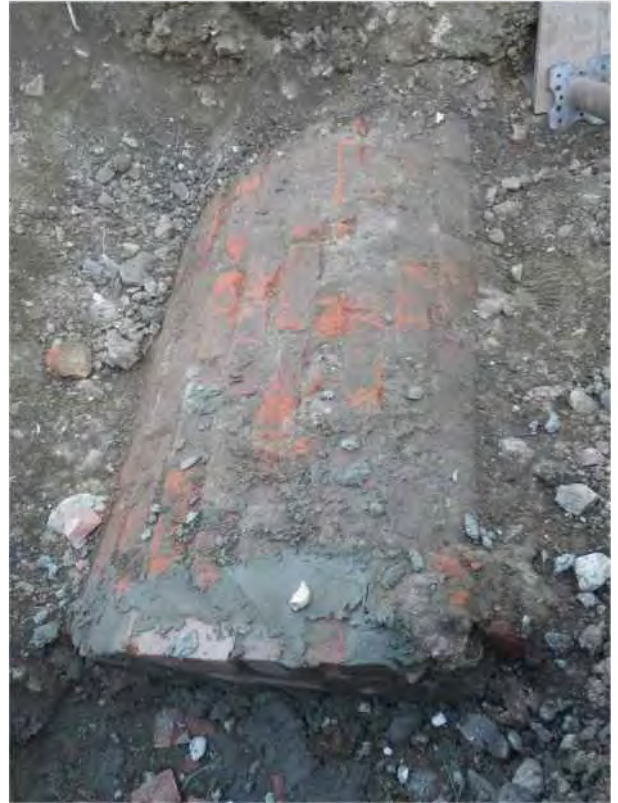
Plate 4: Repair to vaulted tomb 103, looking west
