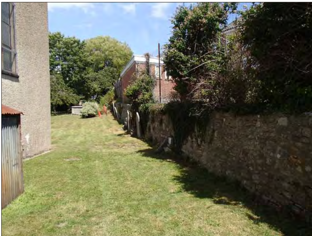
Plate 2: General view of southeast boundary wall, prior to works, looking northeast
