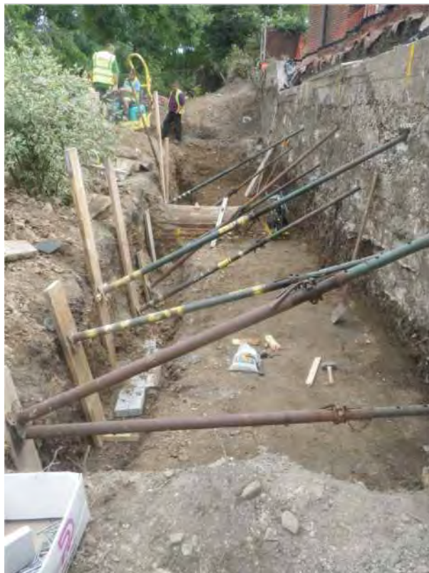
Plate 5: View of excavated trench, looking north
