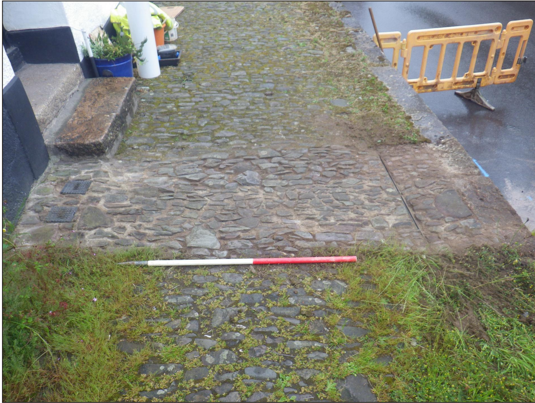
Plate 1: Cobbles cleaned prior to lifting, looking west. Scale 1m
