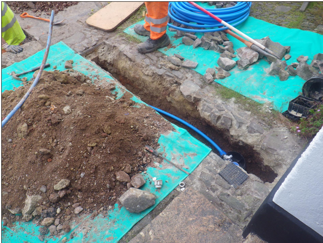
Plate 2: The excavated trench, looking northeast
