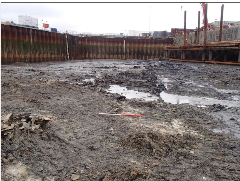
Plate 3: The drained wet basin showing exposed solid bedrock below foreshore silts, view from west (1m scale)
