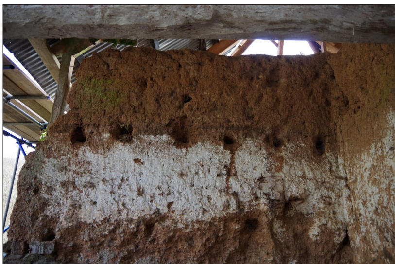
Plate 7: Sockets for the first-floor beams in the east internal wall viewed from the west
