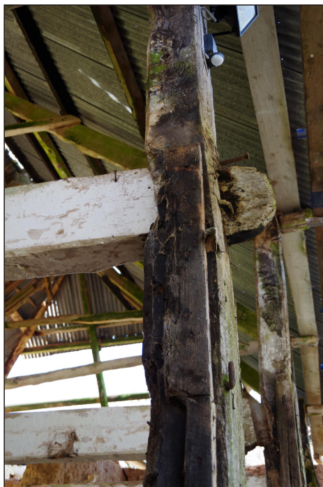
Plate 5: mortice and tenon joint on a first-floor beam and upright viewed from the northeast
