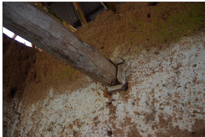
Plate 6: Boards surrounding a first-floor beam in the central cob wall also showing remnants of lime plaster viewed from the southeast
