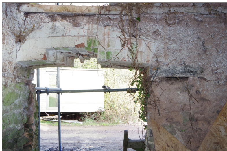
Plate 10: The remains of the wooden lintel in the east room viewed from the south
