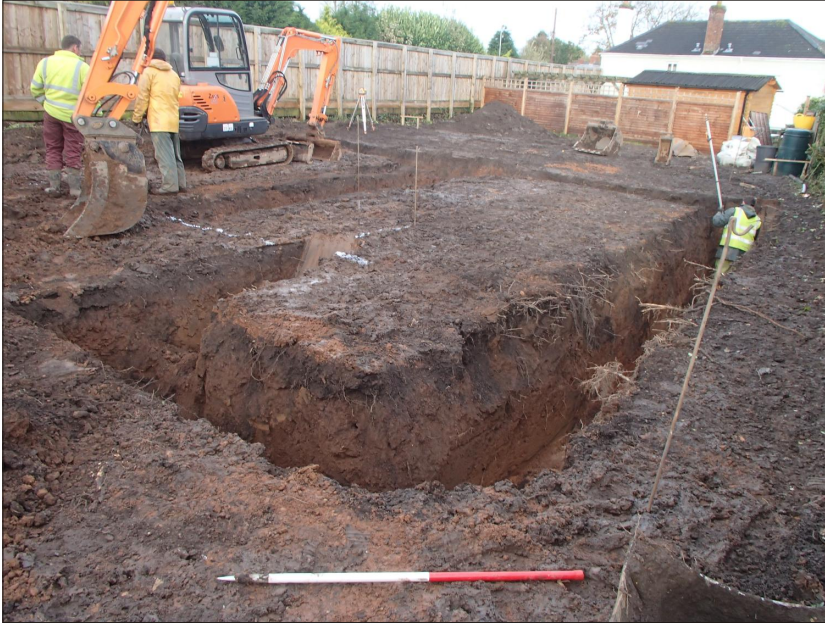
Plate 1: View of house footings looking north (1m scale)
