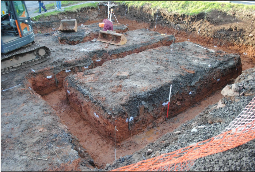
Plate 4: View of garage footings, looking northwest (1m scale)
