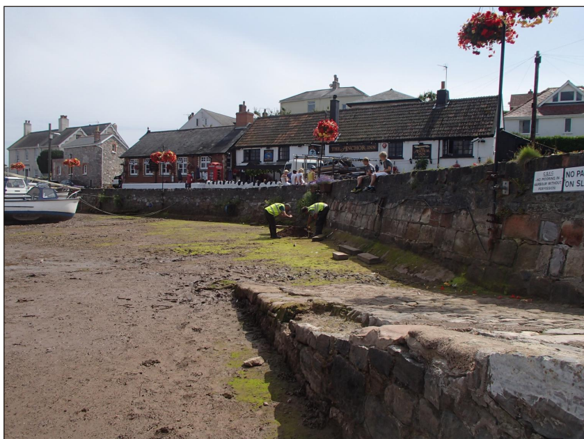
Plate 3: Excavation of test pit 4 in progress, looking south
