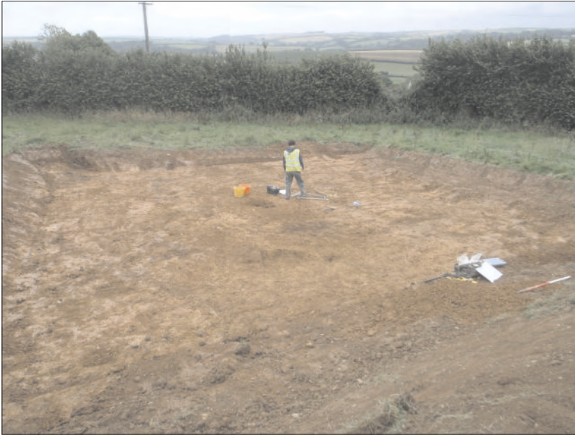
Plate 1: Excavation in progress, looking southeast
