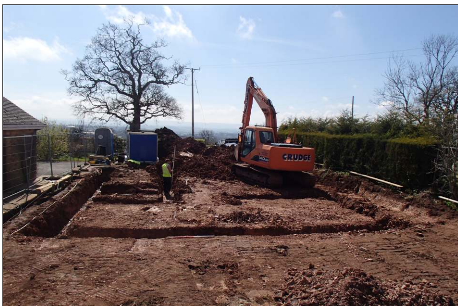
Plate 2: Showing working view of footings trench excavation. Looking southwest
