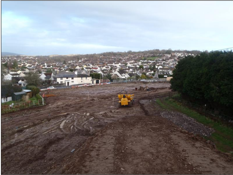
Plate 1: General view of site looking northeast towards Vicarage Hill Road
