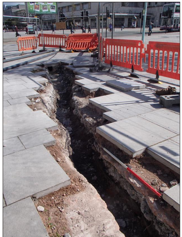
Plate 3: Trench 2, general view, looking north. 1m scale
