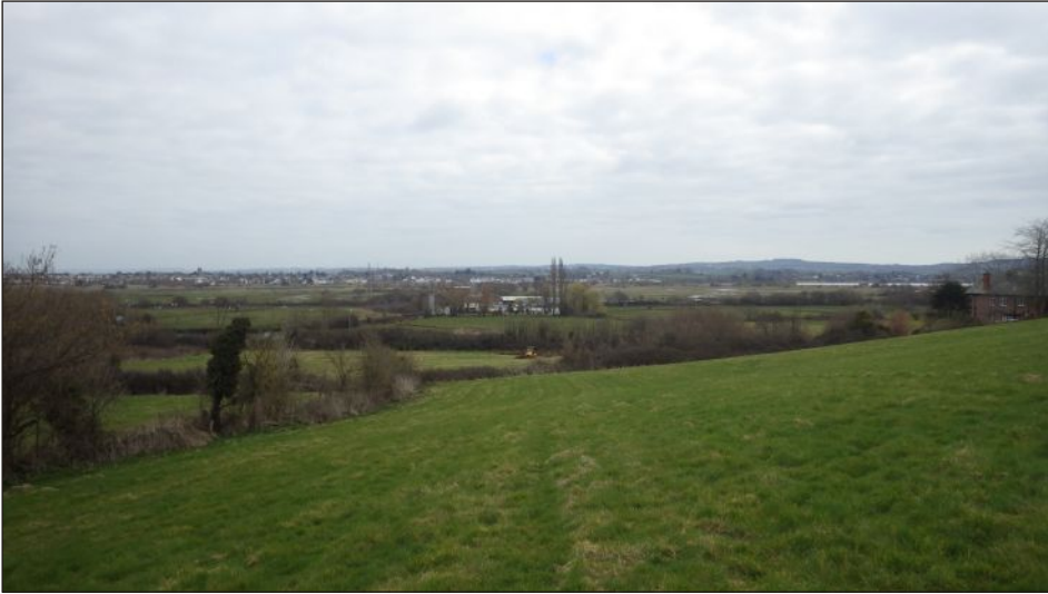
Plate 1: General view of site, looking northeast
