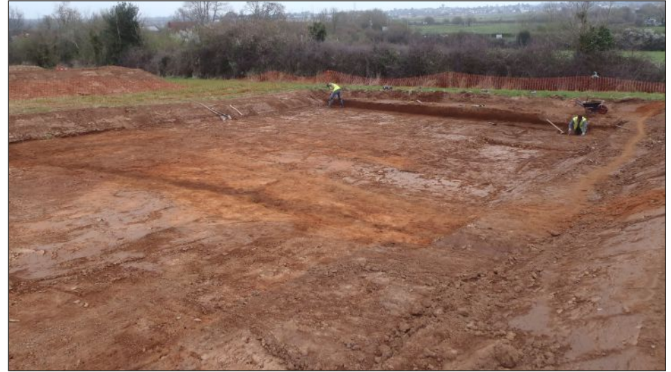
Plate 2: Excavation area in progress, looking north
