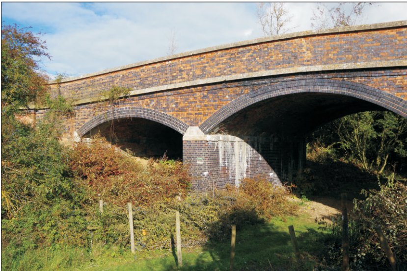
Plate 8: General view of the south elevation, looking northwest
