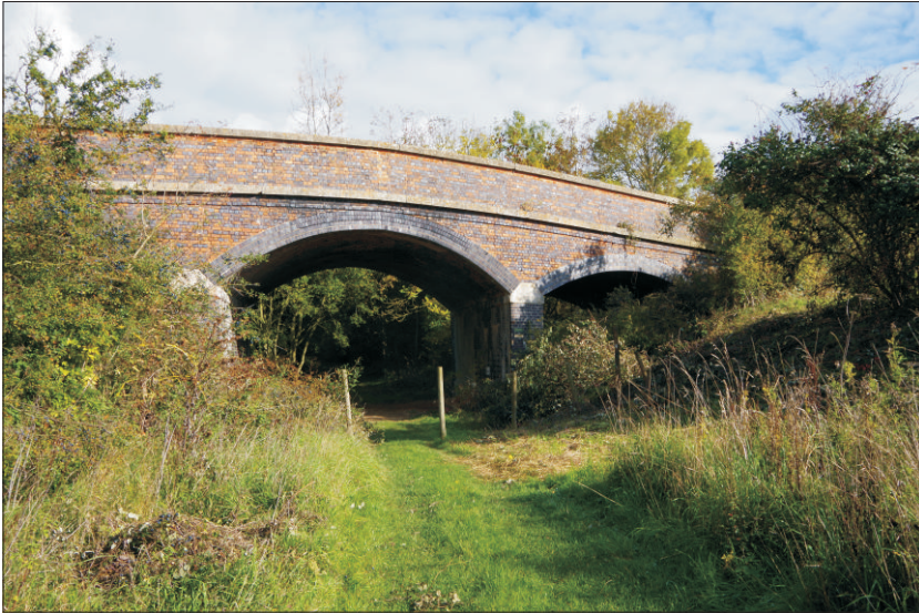
Plate 7: General view of the south elevation, looking north
