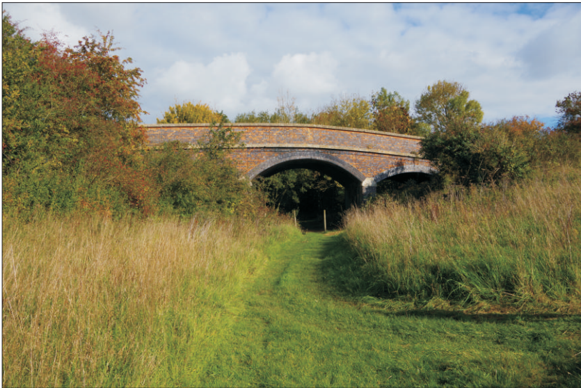
Plate 4: General view of the south elevation, looking north
