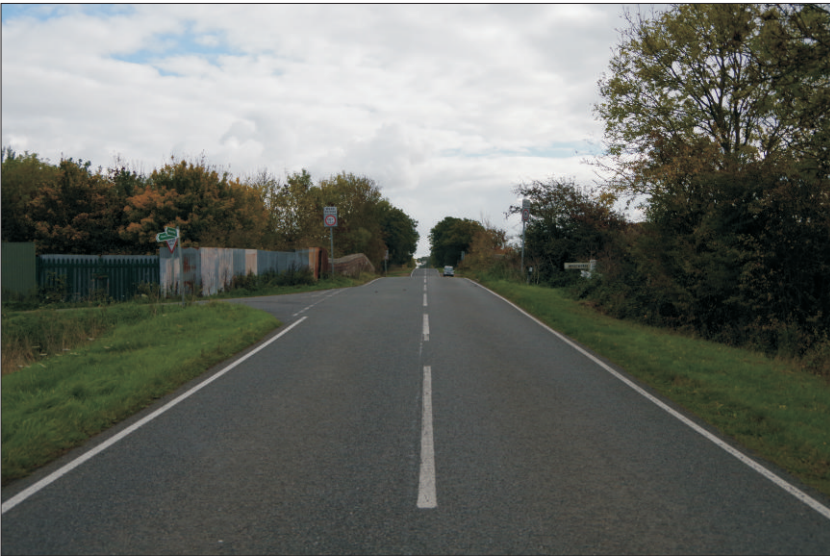
Plate 2: View of the B662 crossing the bridge, looking southeast
