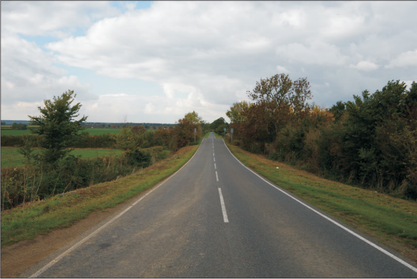
Plate 1: View of the B662 crossing the bridge, looking northwest
