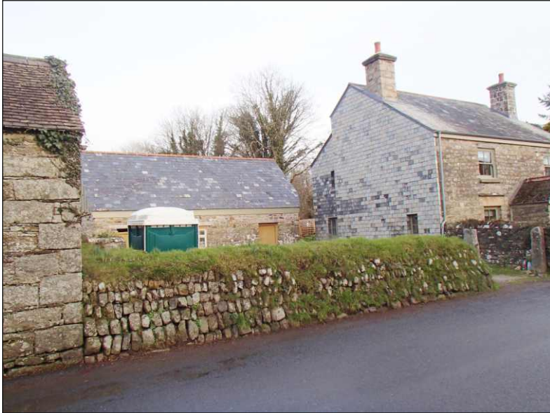
Plate 1: General view of Castle House. Looking north
