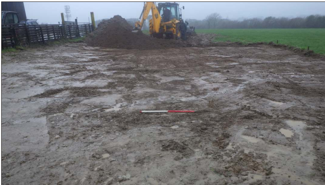
Plate 3: Showing stripped area for Building 2. View to west (scale 1m)
