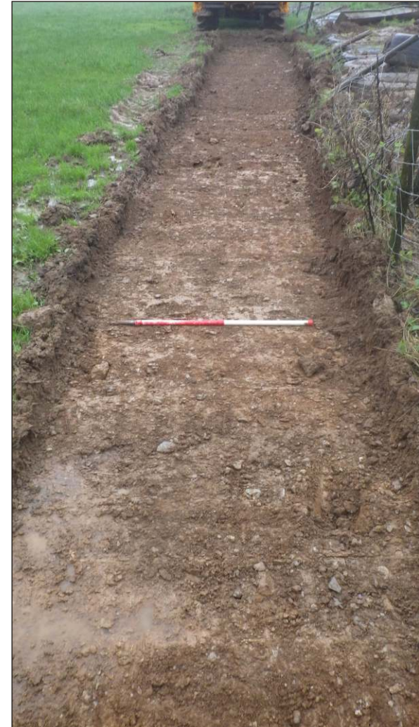
Plate 2: Showing stripped area for Building 1. View to southwest (scale 1m)
