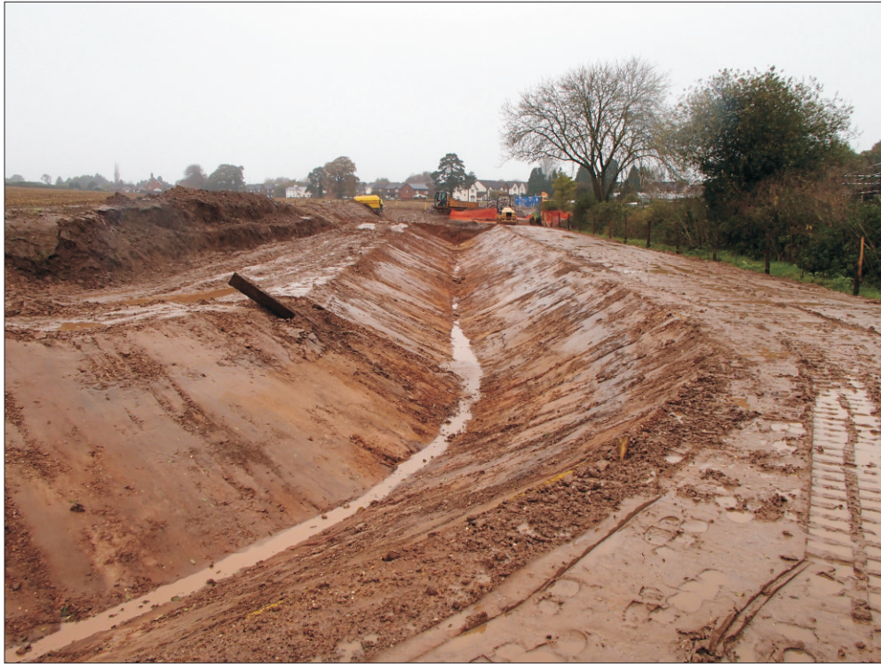
Plate 1: General view of flood alleviation channel, looking NNE
