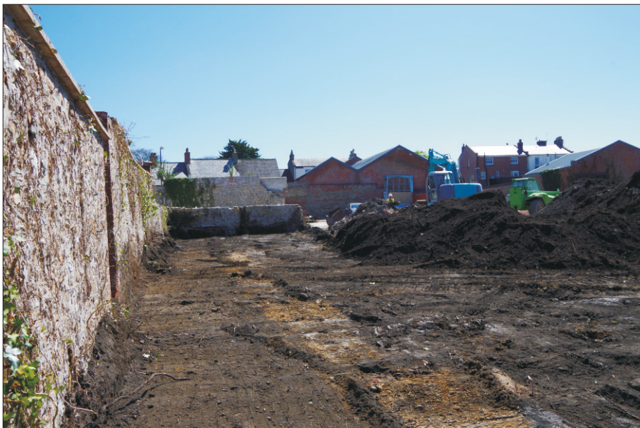
Plate 4: General view of Area 2 after reduction showing path foundation, looking east
