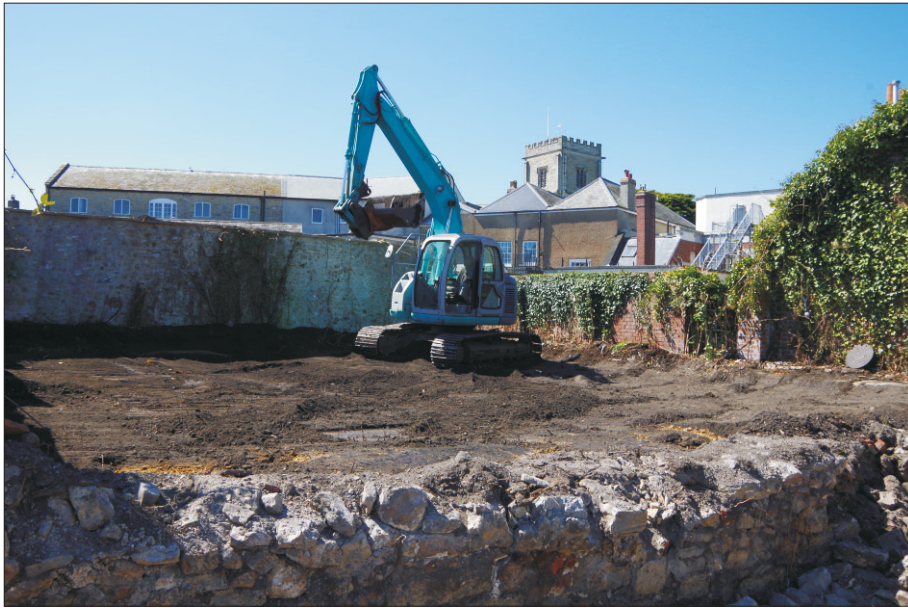
Plate 3: General view of Area 1 after reduction, looking southwest
