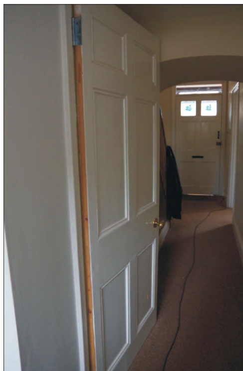
Plate 6: An example of one of the panelled doors with simple moulding
