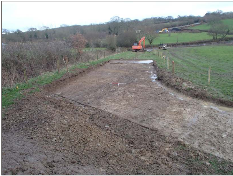
Plate 1: View of north section of Area 1. Looking southeast (scales 2 x 1m)
