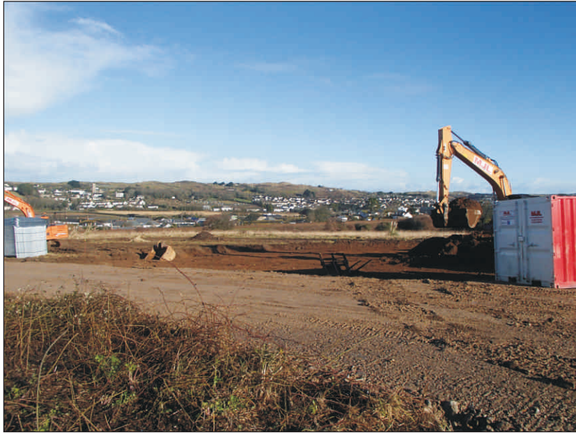
Plate 1: General view of Area A, work in progress, looking northeast
