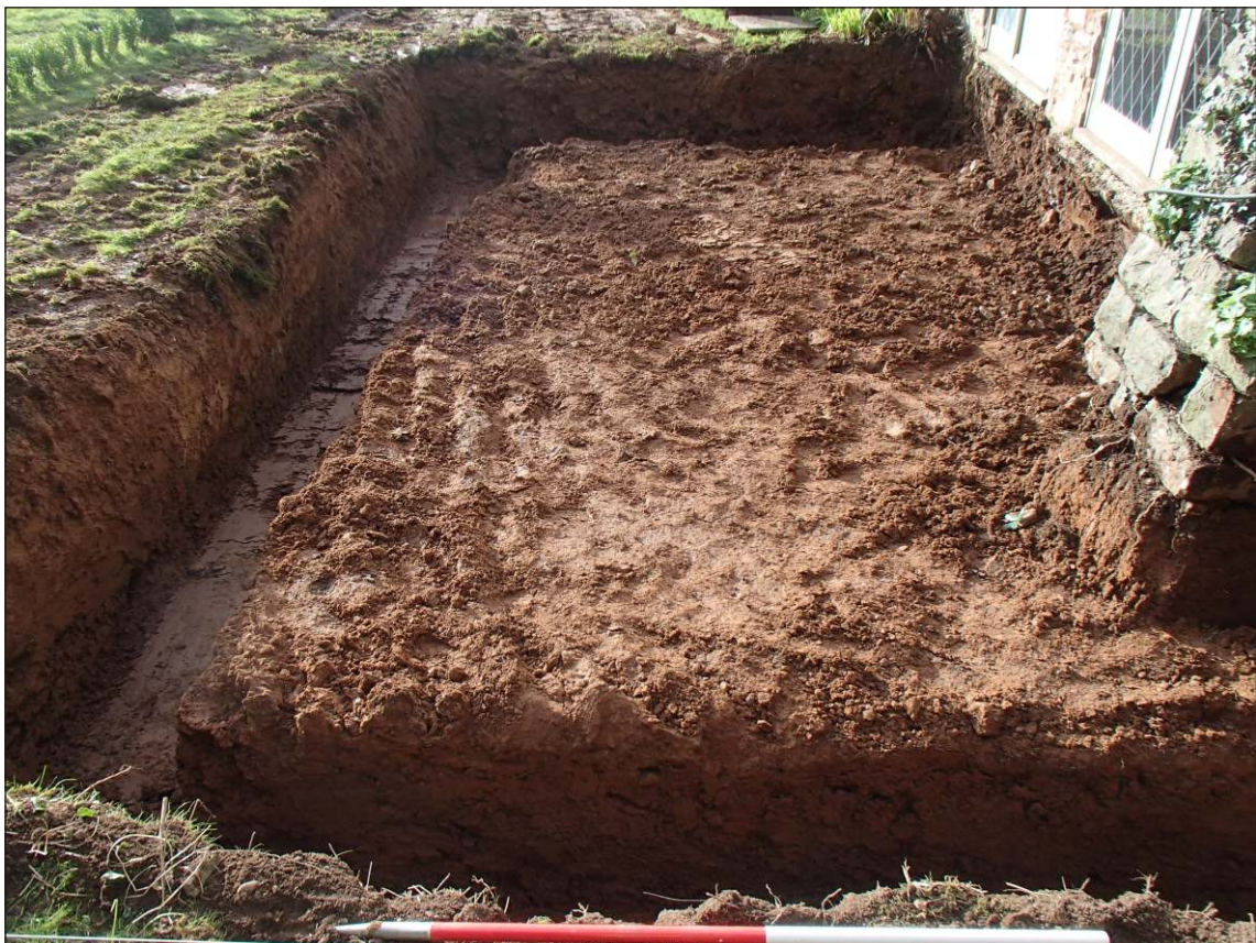
Plate 2: Post-excitation view of foundation trenches, view to southwest (scale 1m)
