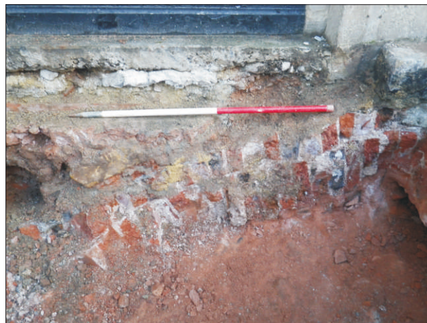
Plate 3: Castle Bow trench, Castle Walk, brick culvert S109, view from the west (scale 1m)
