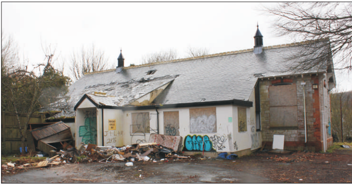
Plate 10: North elevation of Ivycroft, looking southeast (1m scale)
