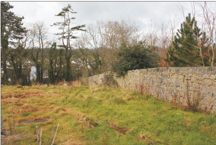
Plate 3: Northern boundary wall, looking west-northwest (1m scale)
