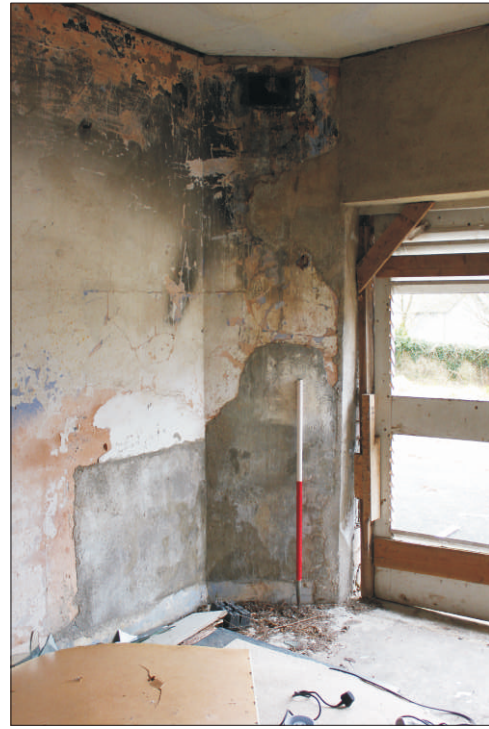
Plate 7: Blocked fireplace in north garage in The Morgue, looking southwest (1m scale)
