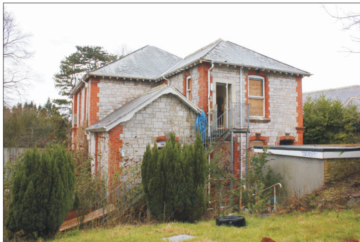
Plate 17: East elevation of The Willows, looking west-northwest
