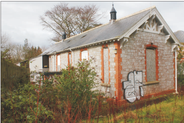
Plate 12: South and east elevations of Ivycroft, looking northwest (1m scale)
