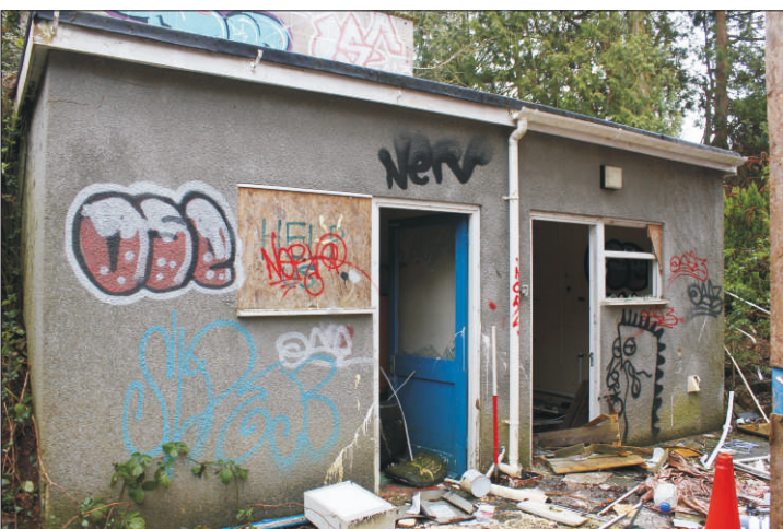
Plate 28: General view of plant building, looking east-southeast (1m scale)
