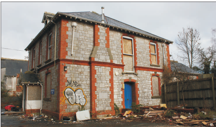
Plate 15: South elevation of The Willows, looking northeast (1m scale)
