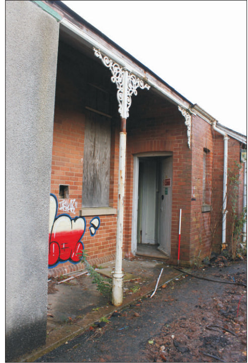
Plate 22: Veranda with decorative iron frame, looking northeast (1m scale)
