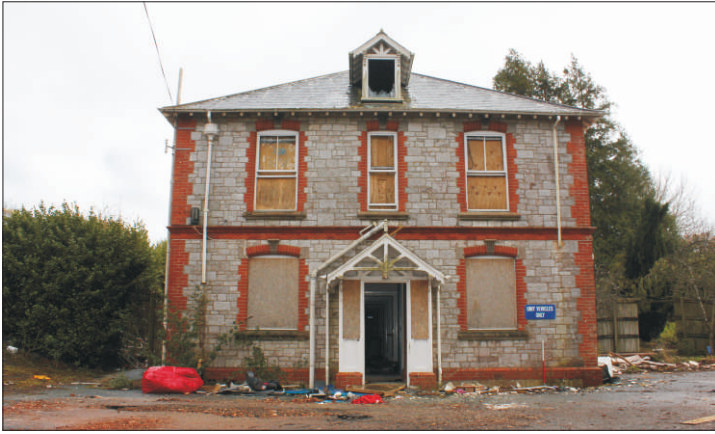
Plate 13: West elevation of The Willows, looking east (1m scale)
