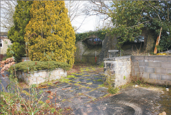
Plate 26: Remains of the Coal Store, looking northeast (1m scale)
