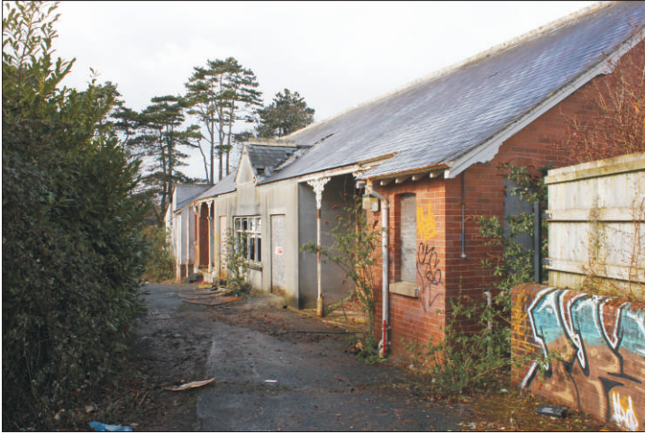
Plate 21: South elevation of the Day Care Unit, looking west-northwest (1m scale)
