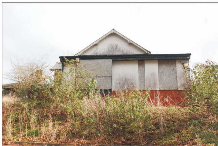
Plate 20: West elevation of the Day Care Unit, looking east (1m scale)
