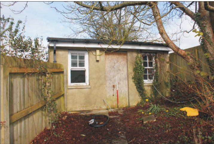
Plate 27: General view of the Gardener's Shed, looking north (1m scale)
