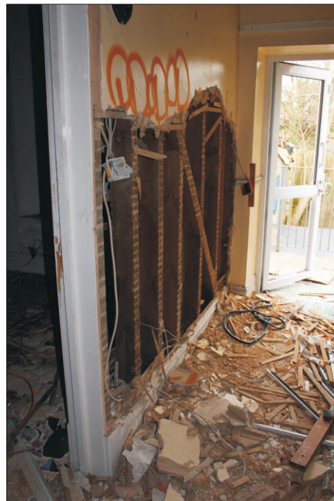
Plate 19: General view of timber-frame partition in The Willows, looking northeast
