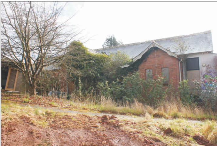
Plate 23: North elevation of the Day Care Unit, looking southeast
