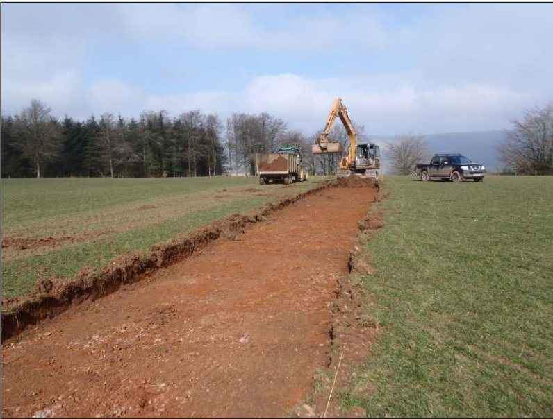
Plate 1: View of trackway strip, looking north in Field 1
