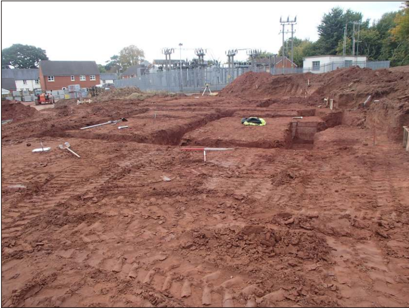
Plate 1: View of site looking west towards electricity substation (scales 2 x 1m)
