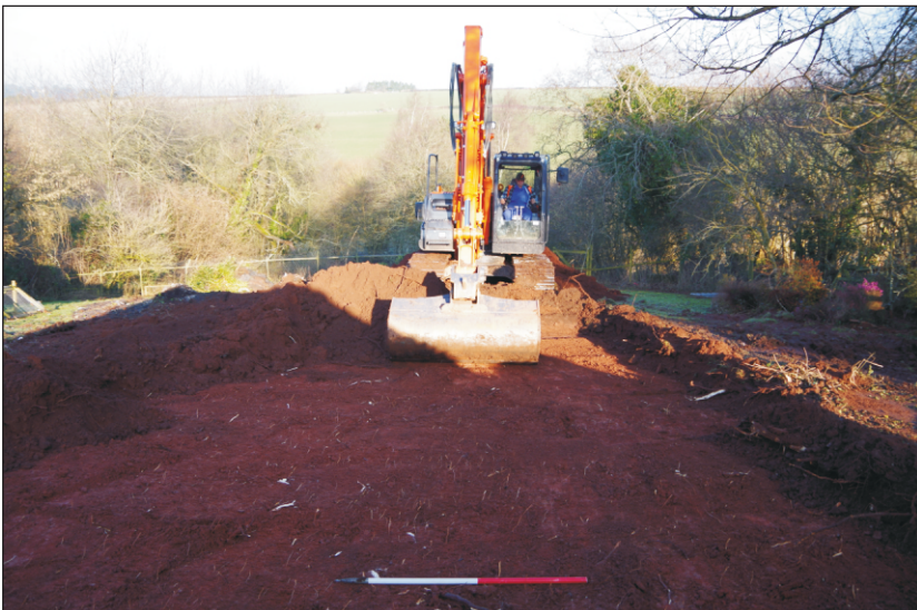
Plate 2: Working view of northwest end of site looking northwest. (1m scale)
