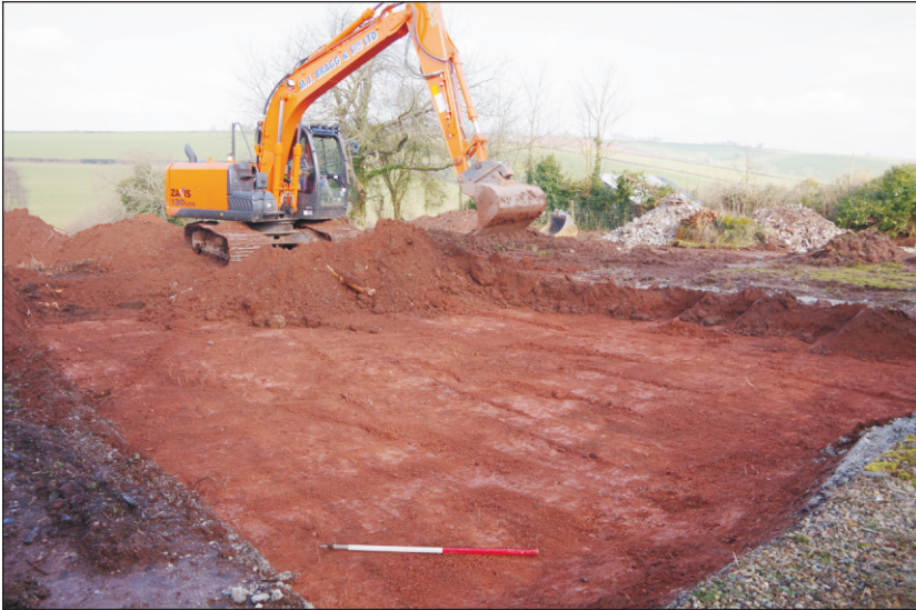
Plate 1: Working view of southeast end of site. looking north-northeast (1m scale)
