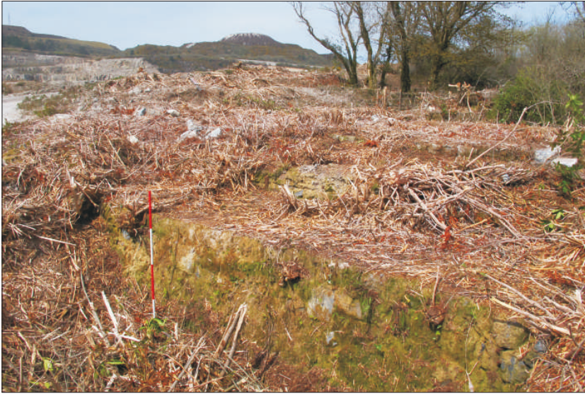
Plate 13: Settling Tank interior north wall, with low walls of the Channel and Mica Drags stepped up behind, from southeast (2m scale)
