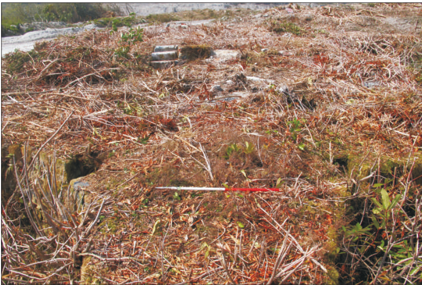
Plate 11: Two inflow recesses for pipes to Round Settling Pit 1 (R) and Round Settling Pit 2 (L), with demolished area and mica drags behind, from east (1m scale)
