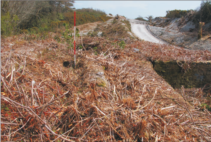
Plate 16: View from west of the Channel (or launder), with scale next to earthenware pipe. The Settling Tank is seen on the right and the mica drag platform on left (2m scale)
