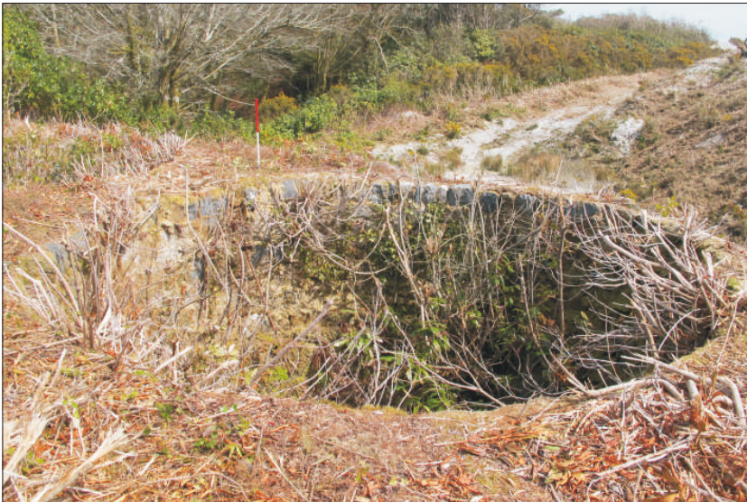
Plate 8: Round Settling Pit 2, overgrown internally, from southwest (1m scale)
