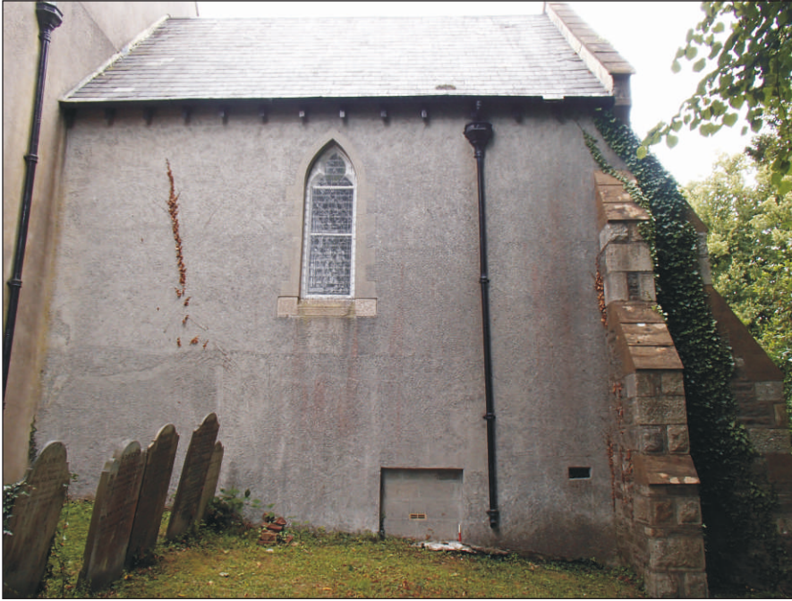
Plate 4: Chancel wall showing blocked access to cellar, looking north (scale 0.2m)
