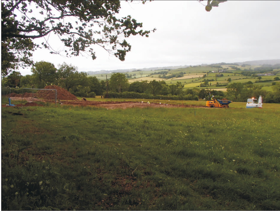
Plate 1: General view of site looking southeast
