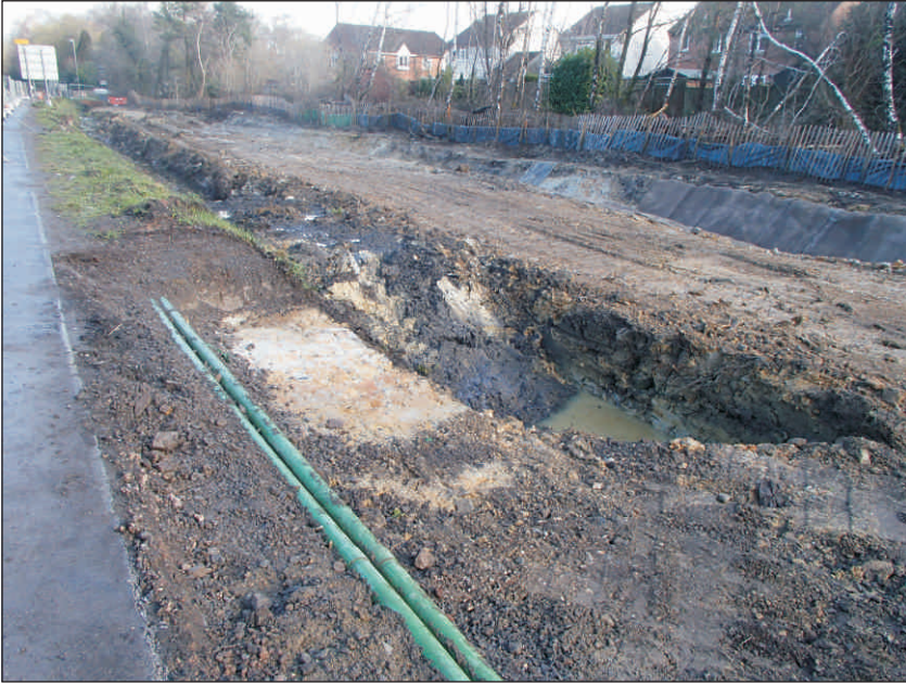
Plate 1: General view of new drainage channel, looking to northwest
