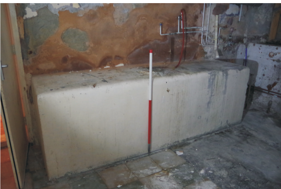
Plate 9: Large concrete slab in the laundry, viewed from the southwest. 1m scale.
