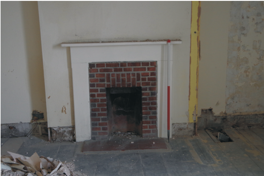
Plate 16: Fireplace in bedroom 6, viewed from the west. 1m scale.
