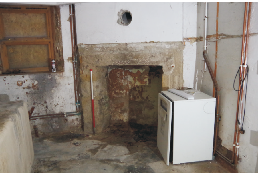
Plate 8: Fireplace in the laundry, viewed from the west. 1m scale.
