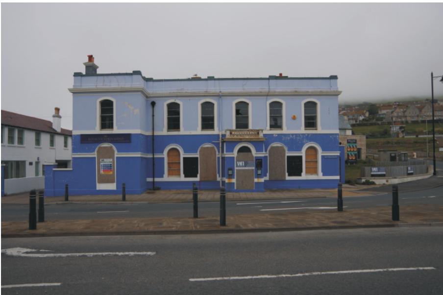
Plate 2: The west elevation, viewed from the west. 1m scale.
