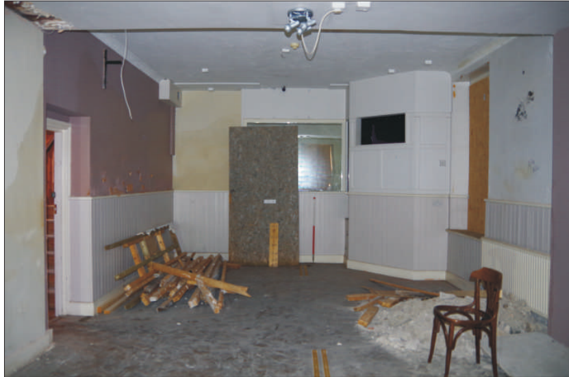
Plate 7: General view of seating area to north, looking east (1m scale)
