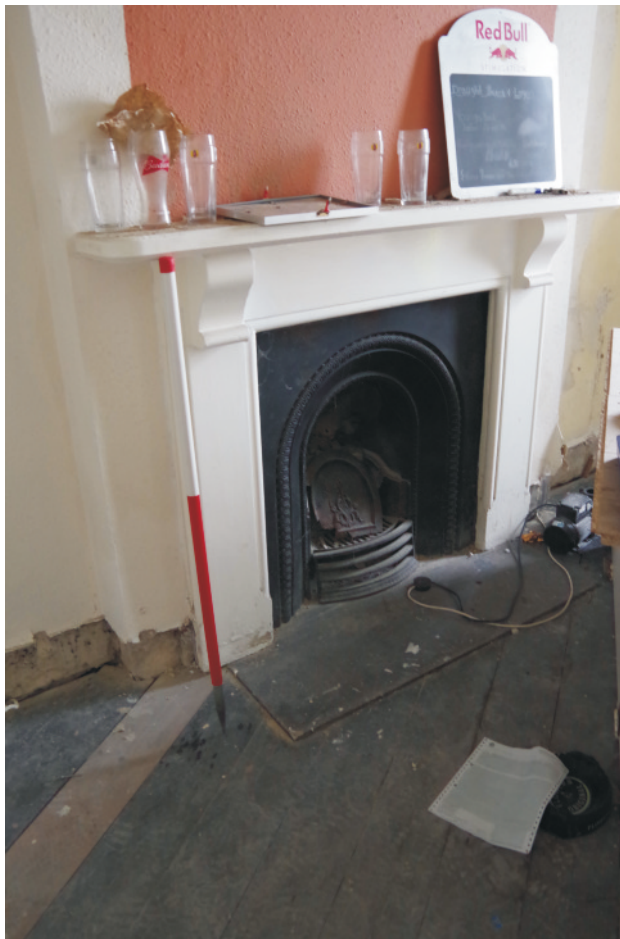
Plate 14: Fireplace in bedroom 4, viewed from the northwest. 1m scale.
