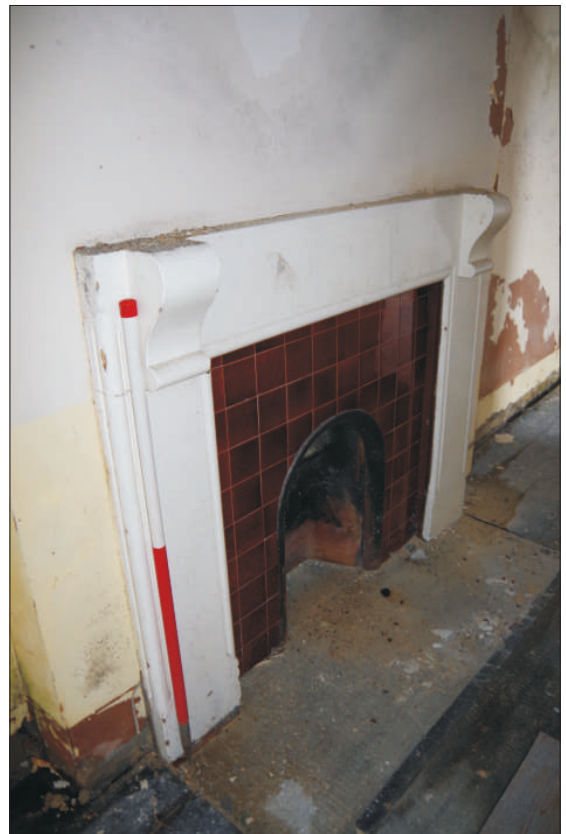
Plate 16: General view of fireplace in corridor to east, looking northwest (1m scale)
