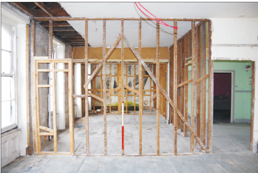
Plate 25: General view of bathrooms 3 and 4 (stud wall between them removed) with bedroom 11 at the back taken from the office, looking north (1m scale)
