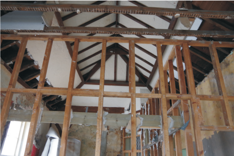
Plate 7: The roof of the northwest block, viewed from the west.
