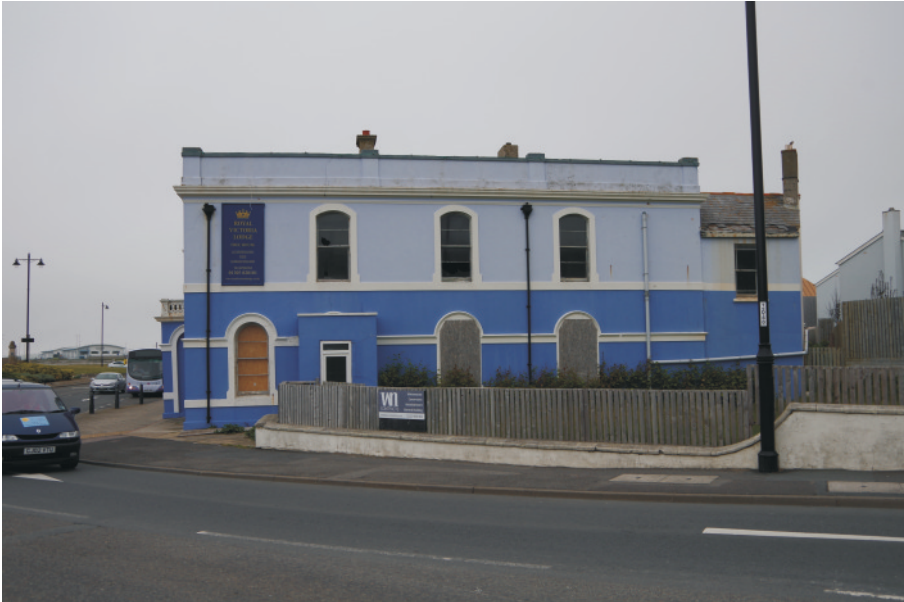
Plate 1: The south elevation, viewed from the south.
