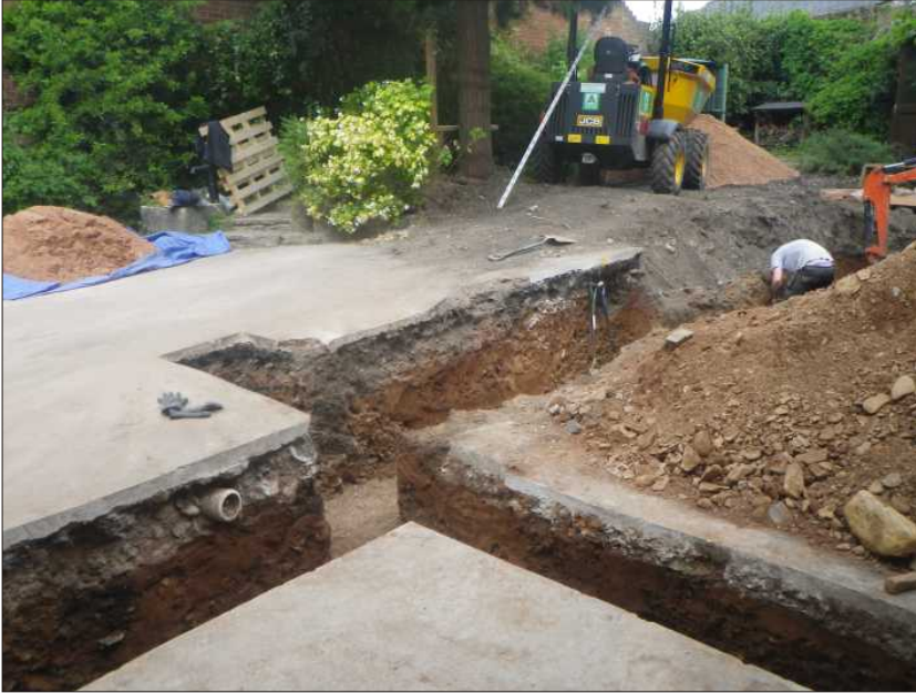
Plate 4: General view of foundation and service trenches, looking north
