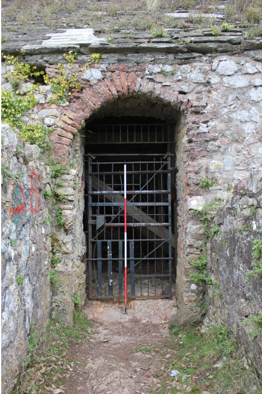
Fig. 8: St Michael's Chapel, Torre doorway, prior to conservation work (2m scale)
