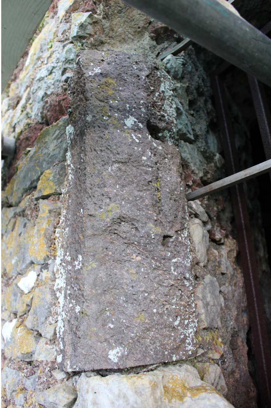
Fig. 12: St Michael's Chapel, Torre higher west window, detail of north jamb
