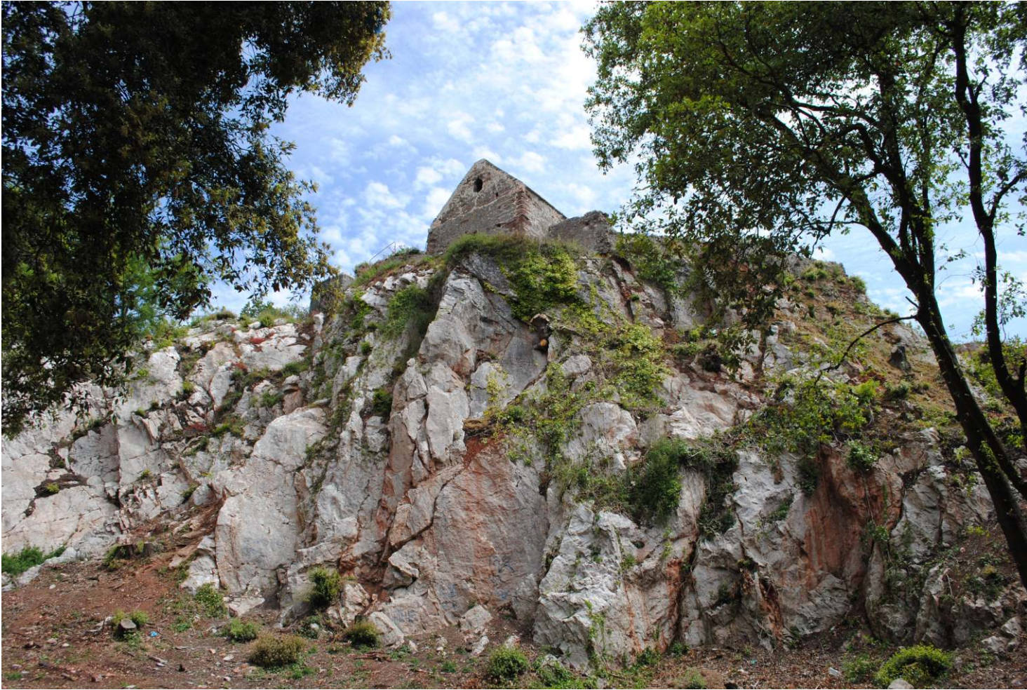
Fig. 4: St Michael's Chapel, Torre following the removal of trees from the limestone quarry. Viewed from the south-west
