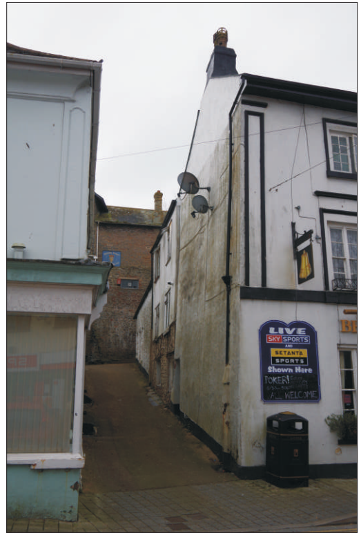
Plate 2: Northeast elevation of the building, looking south-southwest
