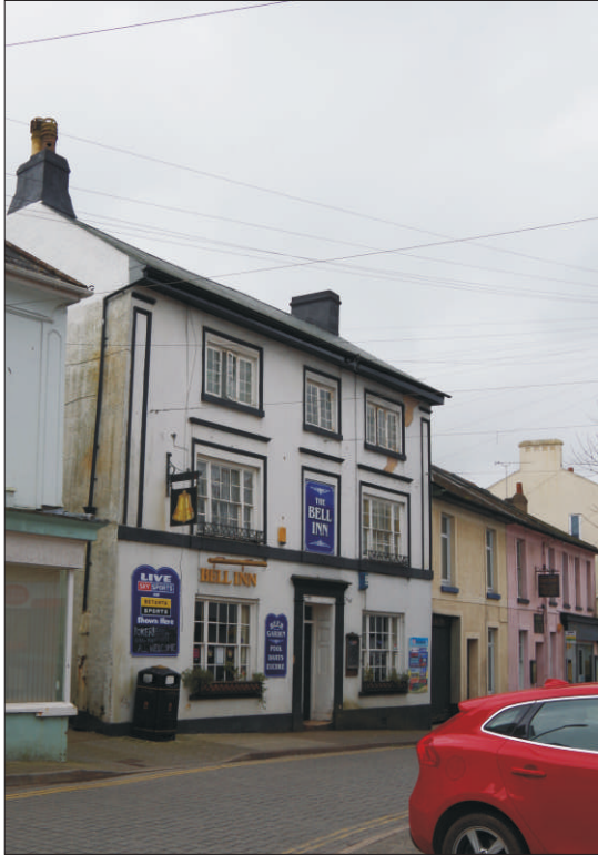
Plate 1: Northwest elevation of front range, looking southwest
