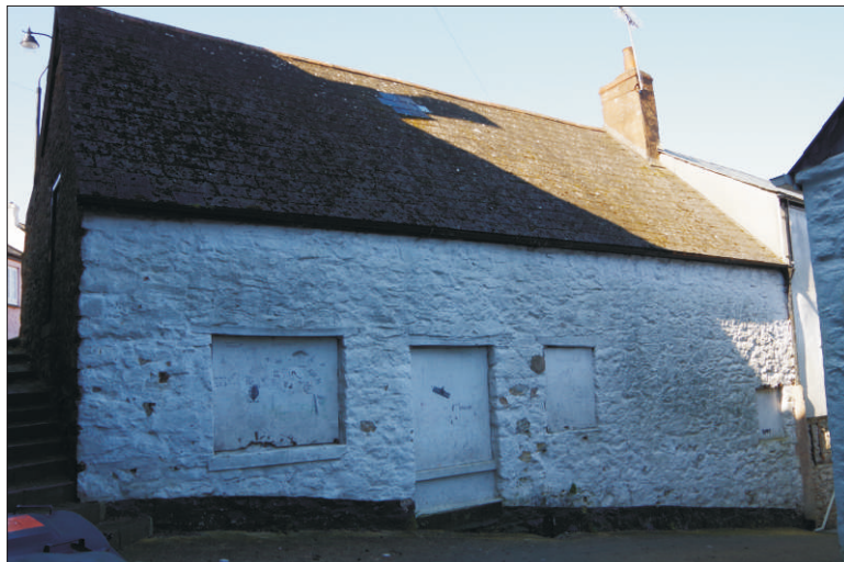
Plate 4: Northeast elevation of the rear range, looking west
