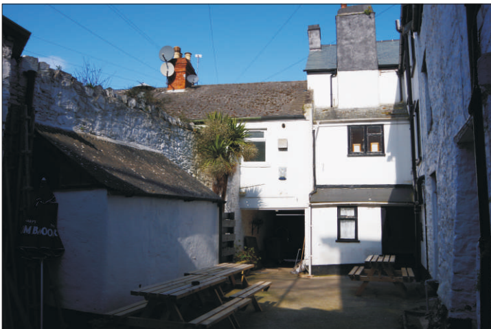
Plate 7: Southeast elevation of the rear range showing the 20th-century extensions, cart entrance and 20th-century outbuilding, looking northwest
