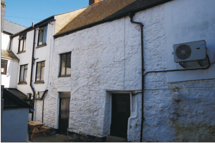
Plate 5: Southwest elevation of the central and rear ranges, looking north
