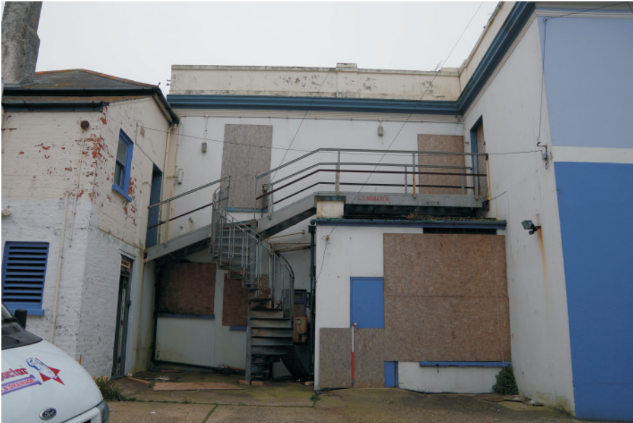
Plate 4: The north elevation of the northern extension, viewed from the north. 1m scale.
