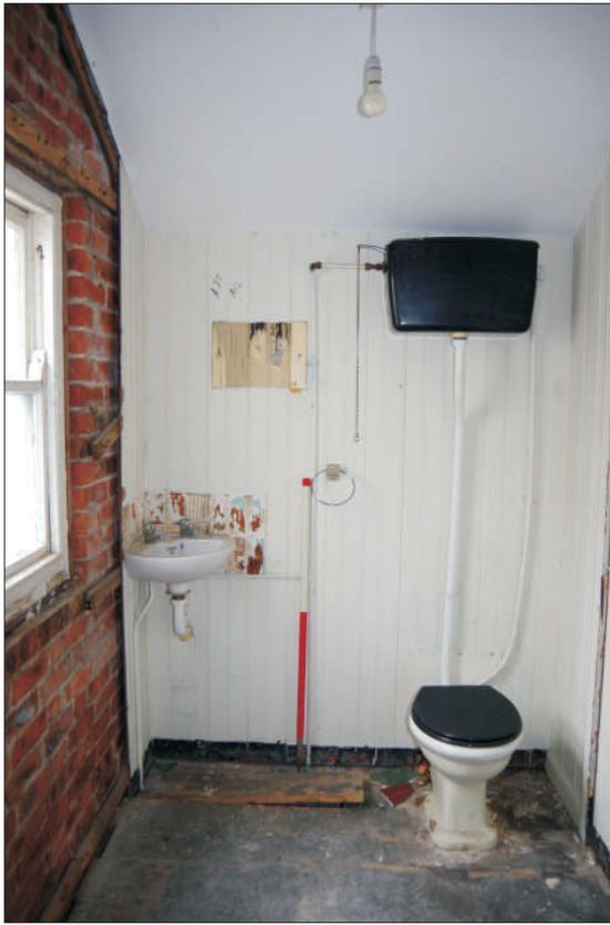
Plate 10: General view of WC, looking north (1m scale)
