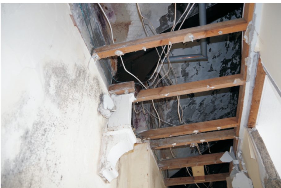
Plate 6: The jointed cruck roof beams on decorative corbels in the east block, viewed from the south.
