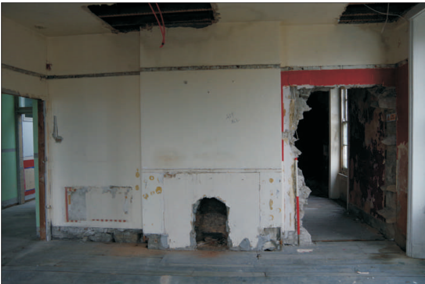
Plate 24: General view of office, looking east (1m scale)
