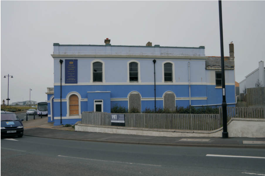
Plate 1: The south elevation, viewed from the south.
