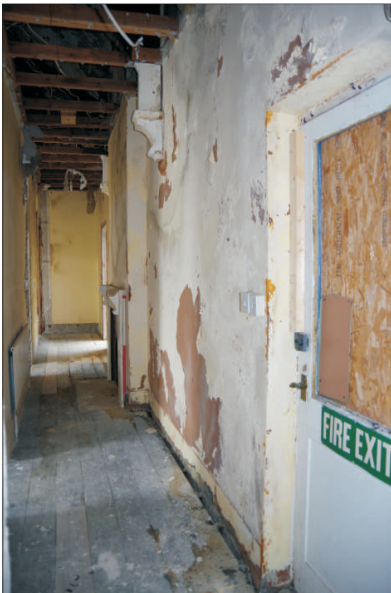
Plate 15: General view of corridor to east, looking south (1m scale)
