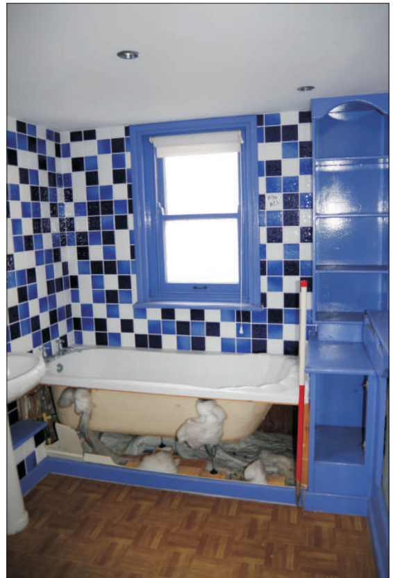
Plate 9: General view of bathroom 1, looking east (1m scale)
