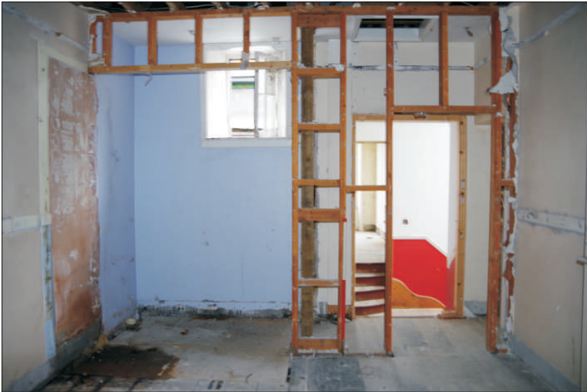
Plate 18: General view of bathroom 2 from bedroom 5, looking south (1m scale)
