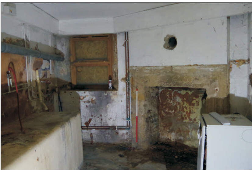
Plate 2: General view of laundry, looking east (1m scale)
