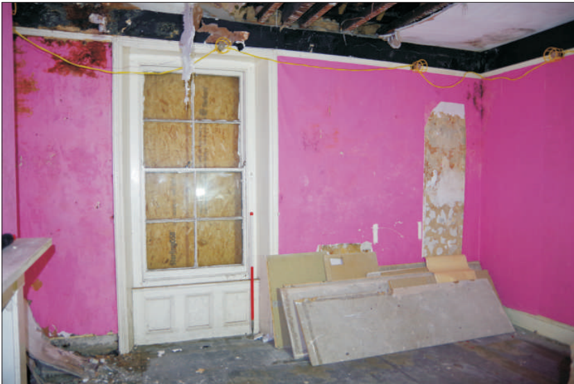
Plate 20: General view of bedroom 7, looking north (1m scale)
