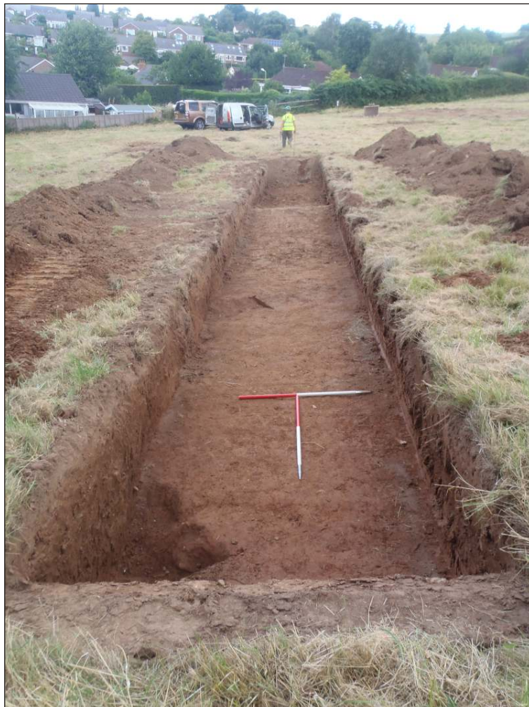
Plate 2: Trench 1, showing ditches F103 and F105, view to northeast (scale 2 x 1m)
