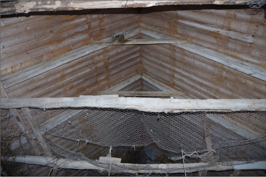
Plate 10: Mill building, roof structure
