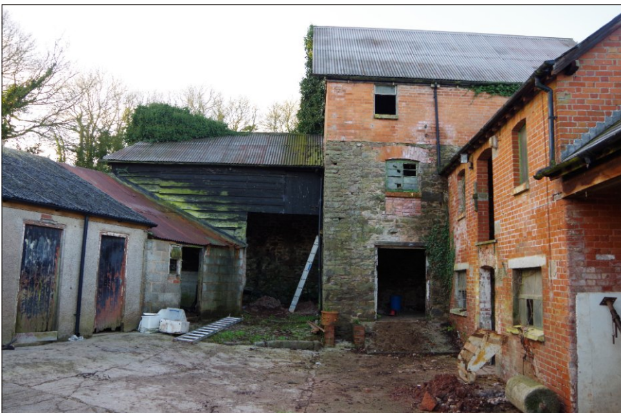
Plate 3: Mill building and east range, north elevations, looking south
