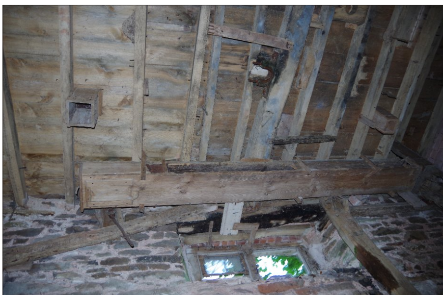
Plate 8: Mill building, base of second floor
