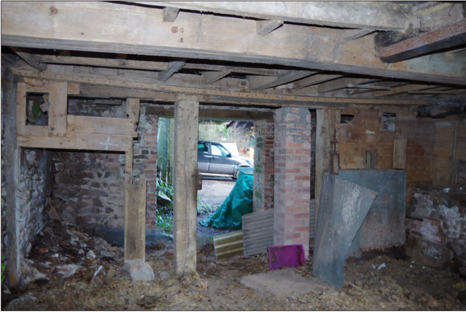
Plate 4: Mill building, ground floor, looking west
