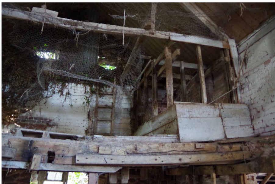
Plate 9: Mill building, second floor from first floor, looking east
