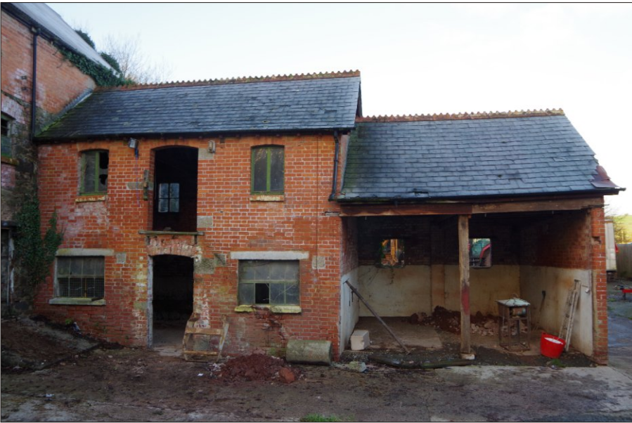
Plate 11: North range and north range extension, looking west
