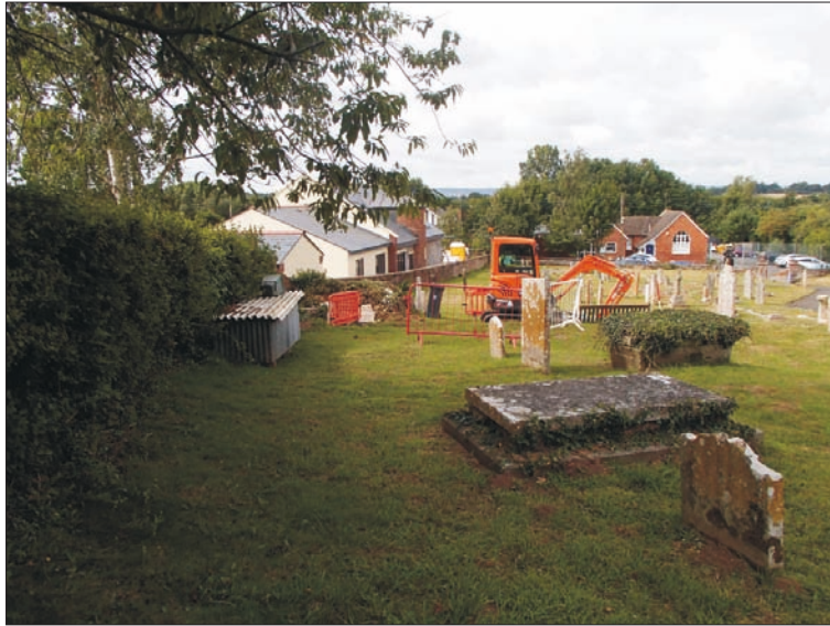
Plate 1: View of churchyard, looking southwest towards excavation area
