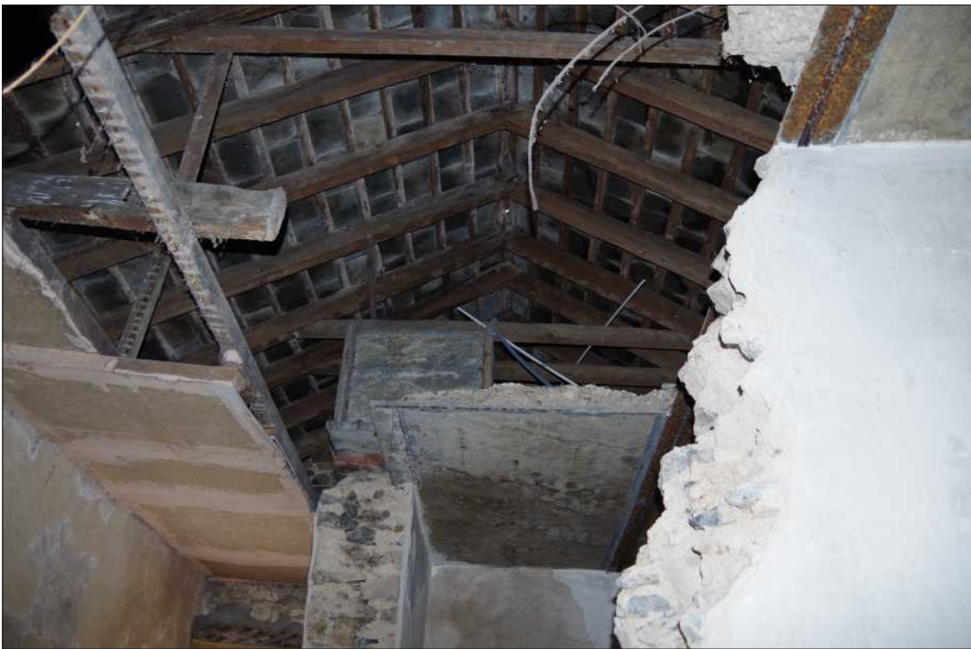
Plate 13: General view of ceiling, water tank and roof, looking south
