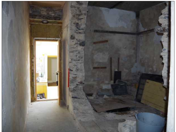
Plate 8: General view of south cell and corridor, looking southwest (1m scale)
