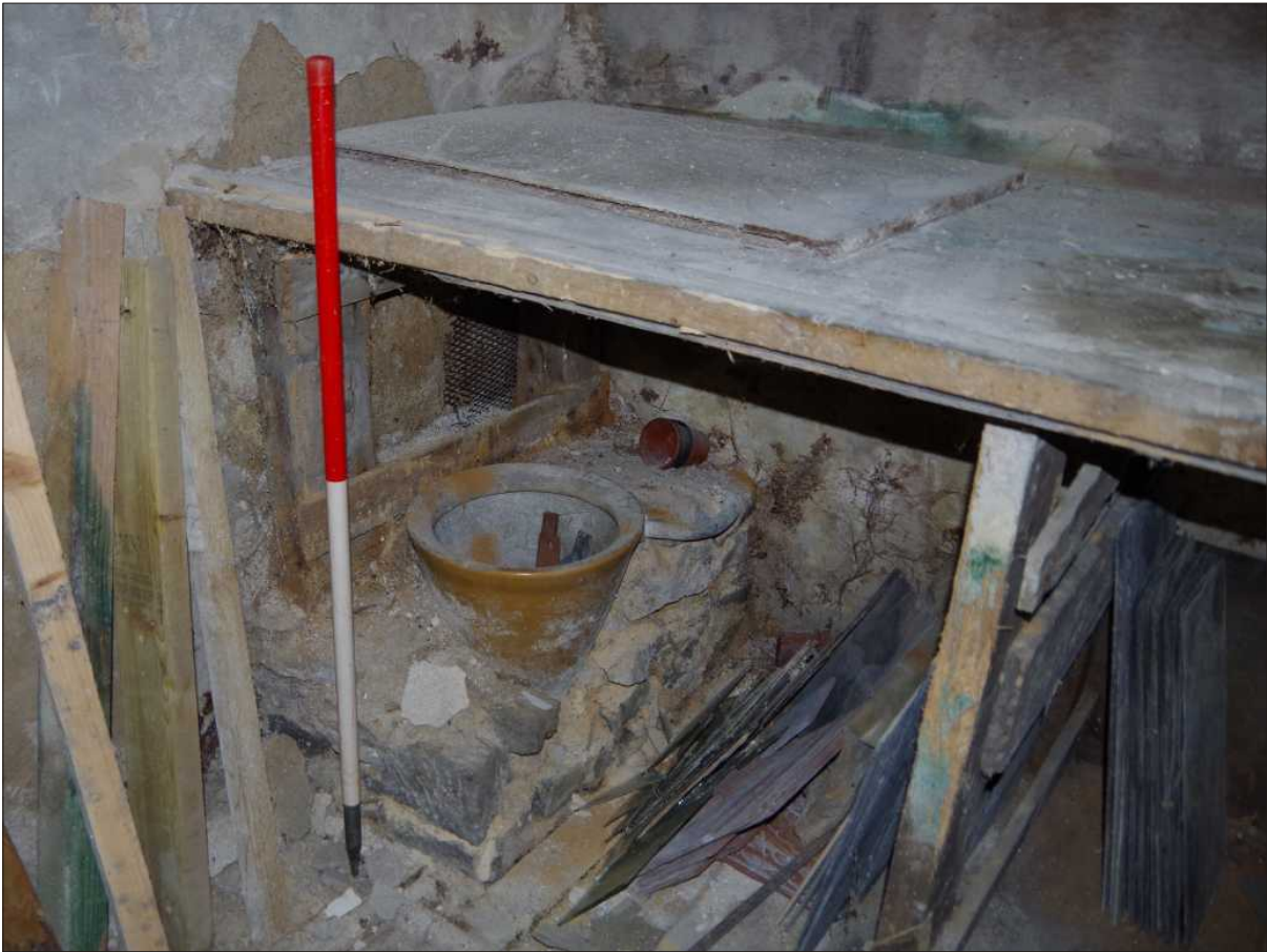
Plate 10: View of rudimentary sanitary facilities, looking northwest (1m scale)
