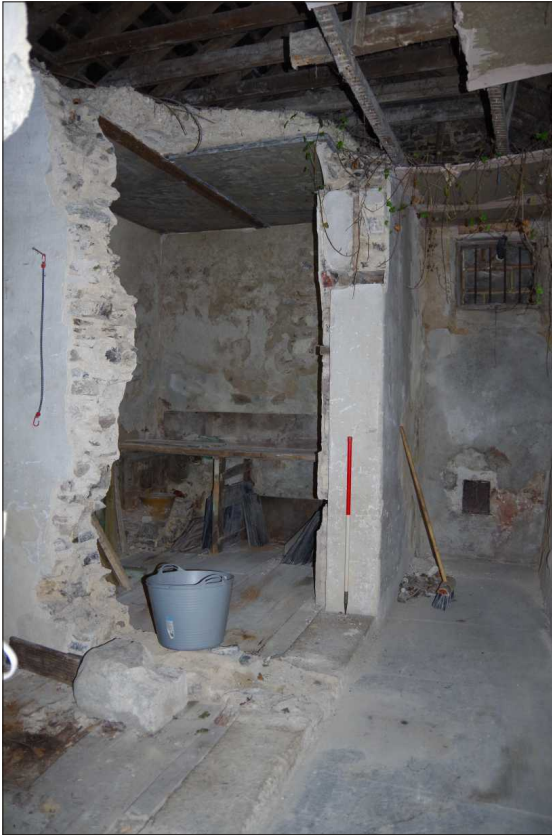
Plate 7: General view of north cell and corridor, looking northwest (1m scale)
