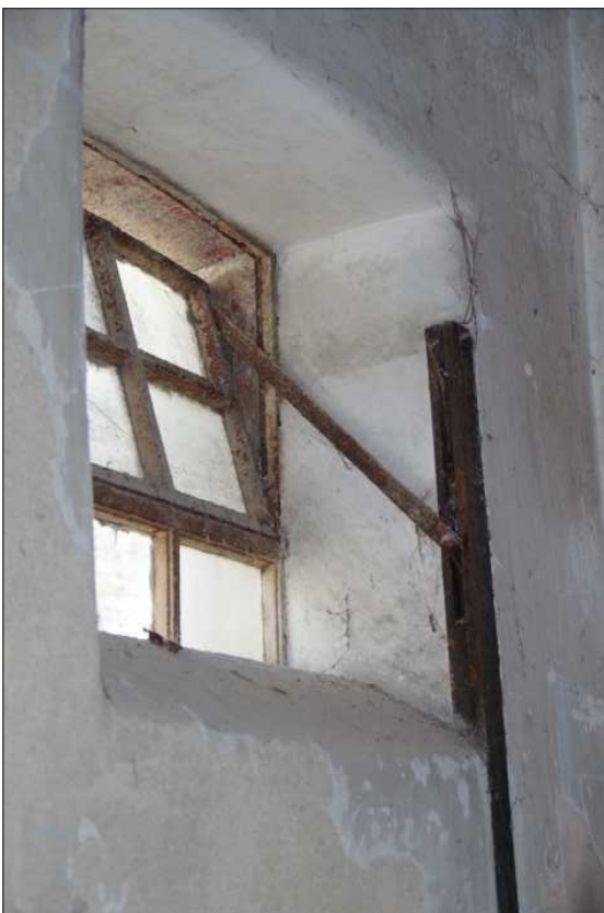
Plate 9: View of metal window mechanism, looking northwest
