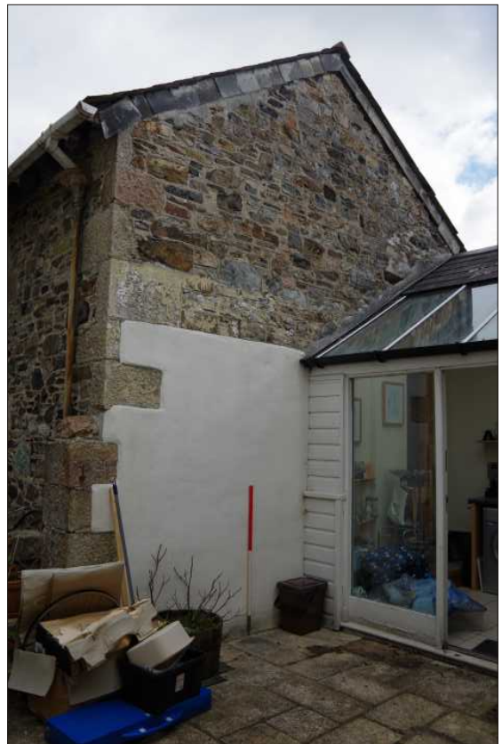
Plate 3: South elevation, looking northeast (1m scale)
