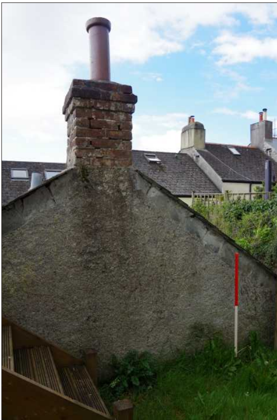
Plate 2: North elevation, looking southwest (1m scale)
