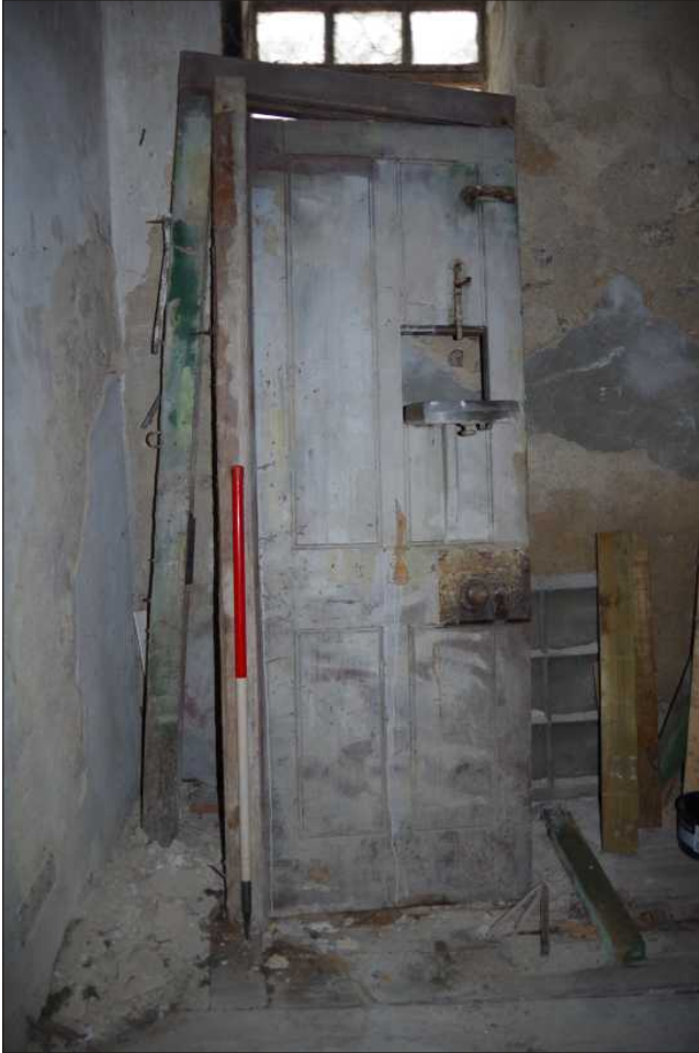
Plate 12: View of cell door, looking west (1m scale)
