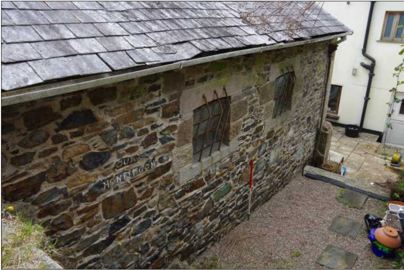
Plate 4: West elevation, looking southeast (1m scale)
