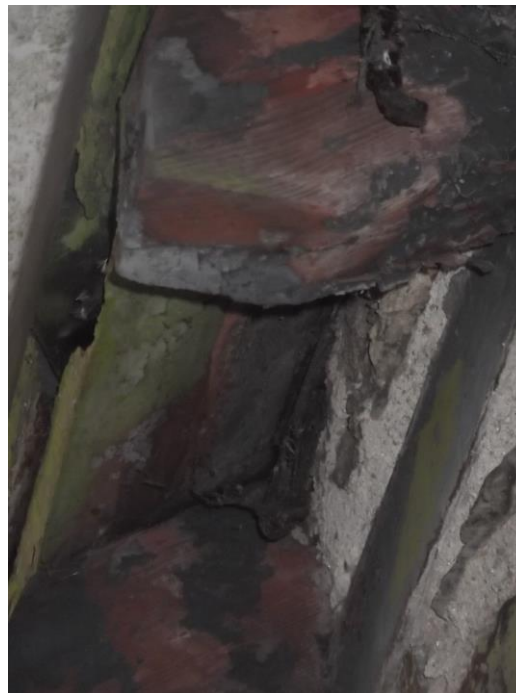
Metal support under eaves
