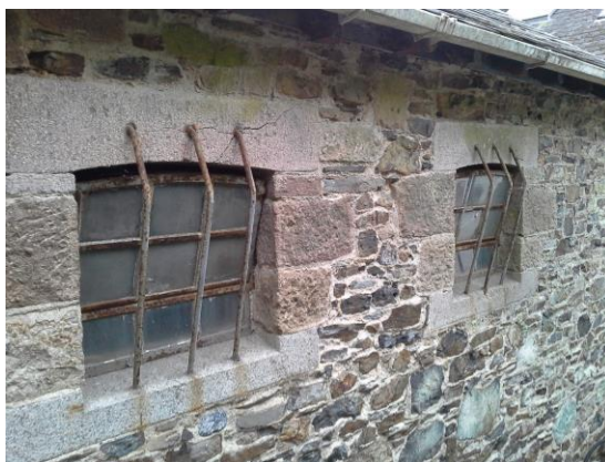
Cell windows showing dog-legged bars
