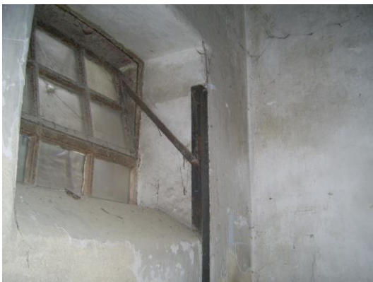
Cell window showing opening mechanism
