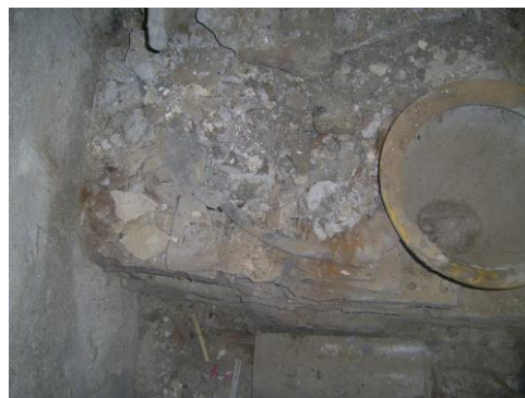
Cell sanitary fitting
