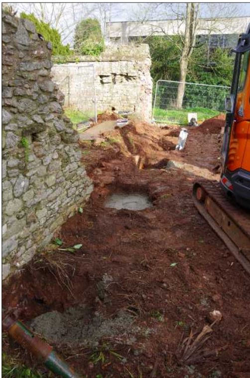
Plate 1: General view of pits after excavation, looking northeast
