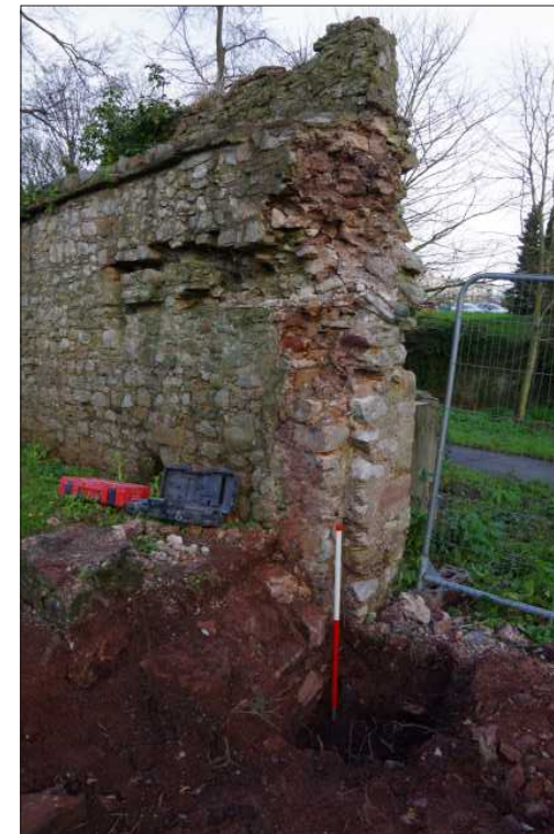
Plate 3: General view of pit 1 and area of doorway in the wall with the surviving rebate in the return wall, looking north (1m scale)
