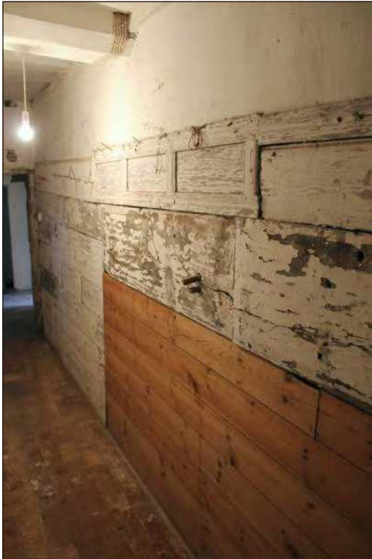
Plate 5: The partition, viewed from the northwest
