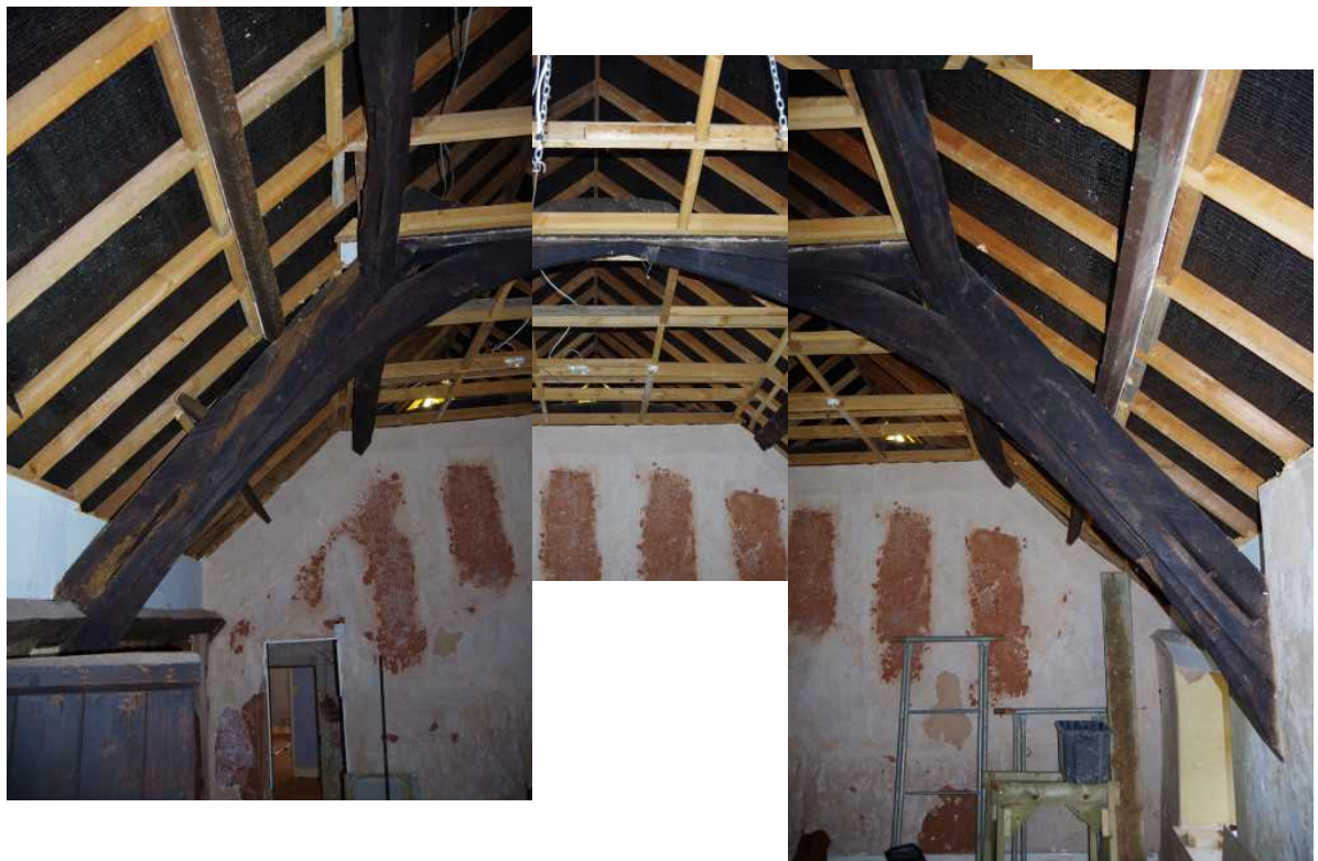
Plate 14: Composite photo of the roof truss, looking east
