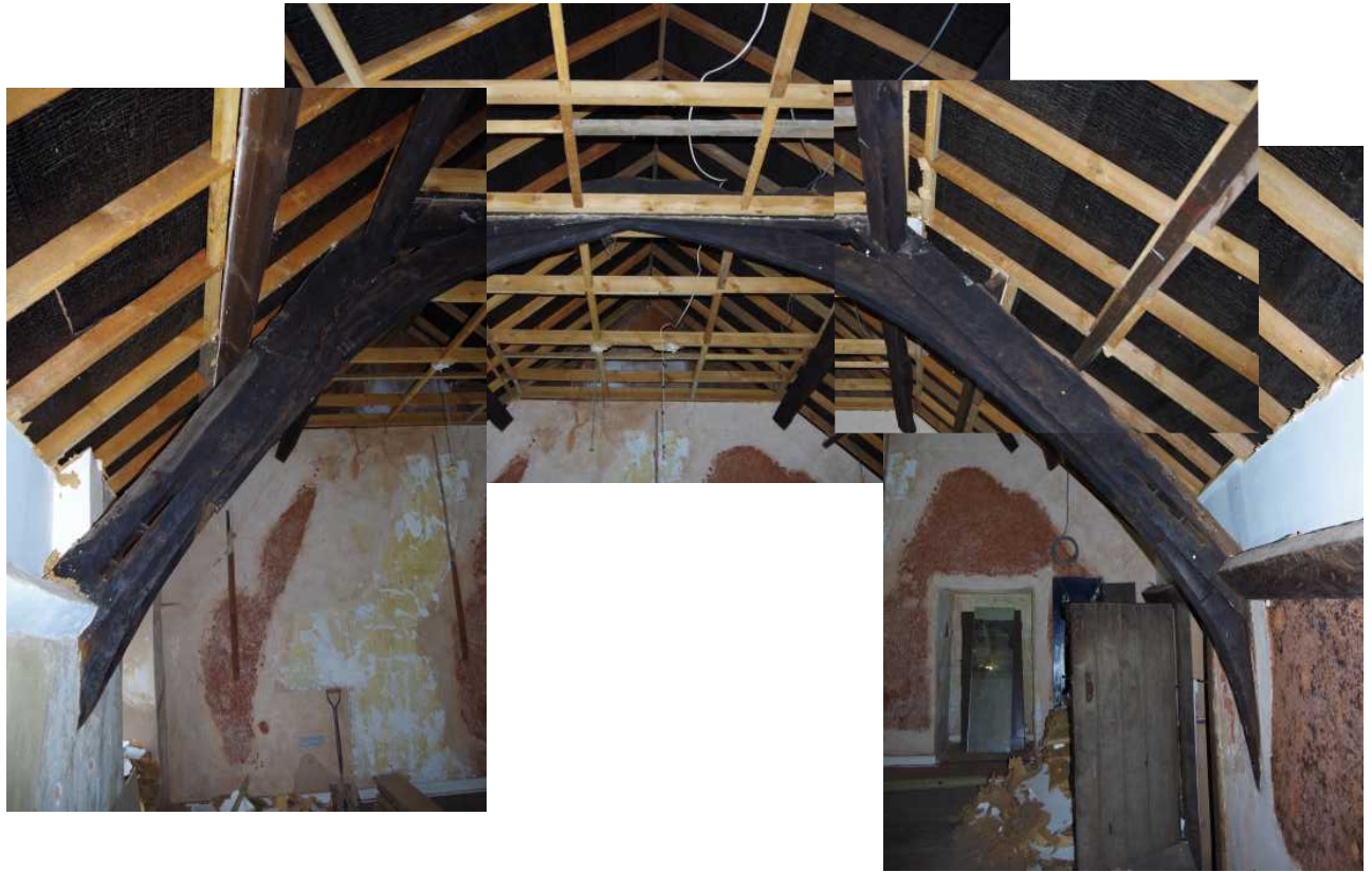
Plate 13: Composite photo of the roof truss, looking west
