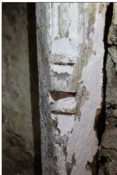
Plate 4: Detail of a stop on the corridor doorframe, viewed from the southeast
