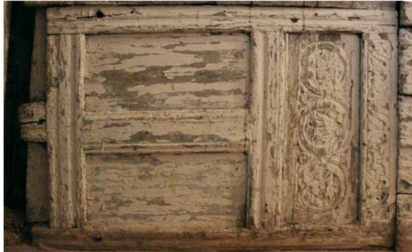
Plate 8: Panel 9, viewed from the north
