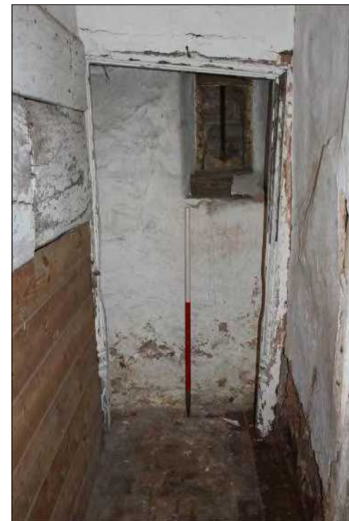
Plate 3: The blocked doorway at the west end of the corridor showing the 17th-century doorframe, viewed from the east. 1m scale
